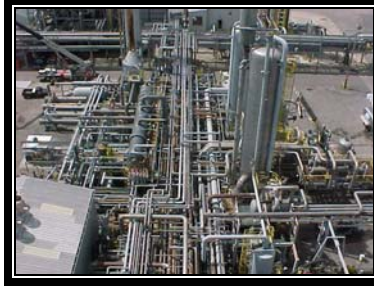
Equipment Covered Lead-Based Coatings
