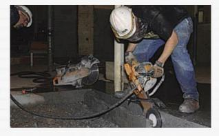
In addition to all of our major sawing equipment, we also have many gas & propane-powered handheld devices such as chainsaws, ring saws and core drills. These hand-held saws and drills allow us to cut and drill penetrations that are not accessible with our larger equipment.
