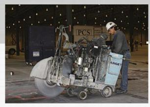
Slab sawing is performed on level and flat concrete surfaces. Using circular diamond blades up to 42 inches in diameter, most common applications include penetrations for ducts, elevators, stairwells, machine pads or to cut trenches for channels or plumbing. It is also utilized by PCS, Inc. in support of demolition services.
