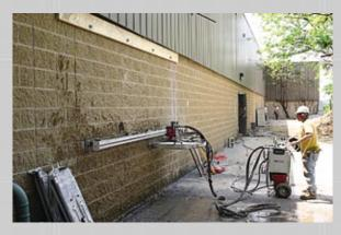
The track-mounted saw is a fast and efficient method of forming large openings. Wall or track saws use a circular blade on a track-mounted machine. The track saw is attached to walls or steep tilts that will not permit the use of floor saws. This method of sawing is preferred for creating defined dimensional door, vent and window openings.
