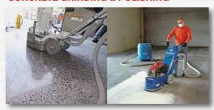
Our state-of-the-art grinding and polishing machines are versatile tools for a wide range of surface preparation jobs. Our low-noise concrete grinding equipment is dust-free which is advantageous when working in environmentally sensitive buildings or industrial facilities. For decorative concrete applications, we can use the same machines to polish concrete to a high shine or to restore old slabs for architectural finishes.
