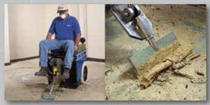
Our ride-on scraping machines have made flooring removal and removal of other materials much easier, faster and more effective. With our fleet of propane, electric and battery-powered machines, we have significantly increased our removal rates and bolstered our productivity on every project that they have been utilized on. Using a variety of scraping blades or teeth, our machines are capable of removing the following flooring applications:
