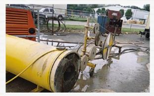
A diamond-encrusted wire is used to perform diamond wire sawing. The precision cutting resulting from diamond wire sawing makes it a superior method if a precise penetration is desired. Since no concrete structure or cross-section is too large to cut, wire sawing is used where other cutting methods are impractical.
