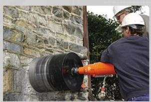
Our powerful high-torque drilling machines provide the tools needed to penetrate a round hole up to 26 inches in diameter. These machines are ideal for drilling holes in floors, walls and ceilings. Each drill rig is equipped with a concrete anchoring system that can be used to drill through concrete, brick, block or stone.
