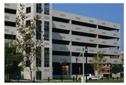
vertical circulation up and down the facility. The garage is directed connected to the adjacent "E-1" Building through two stair elevator cores at both ends of the garage. These stair / elevator towers serve both the building and the garage. Additionally, a third stair elevator tower is provided at Bulldog Way Street. The garage is a six level garage designed with the capacity of an added future floor. O&S Associates provided architectural, structural, and MEP Design services for this project.
