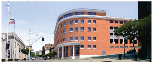
**O&S Associates** with GRAD Associates designed the 600 car Buena Vista parking structure for the City of Yonkers. This self-park, public parking facility was designed with a long span (column free parking bays) and an attractive exterior façade, which blended into the historic waterfront area in Yonkers. The \$9.0 million dollar Buena Vista parking facility was also designed to meet the budgetary constraints of the City.
