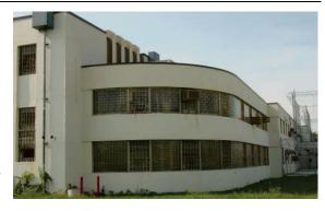
brick masonry, the addition of epoxy grouted masonry ties, tuck-pointing of deteriorated mortar joints, caulking of selected windows and installation of temporary sidewalk protection/bridge. The total cost of the façade repair and roof replacement work was approximately \$6.0M. This was a multi-year phased project.
