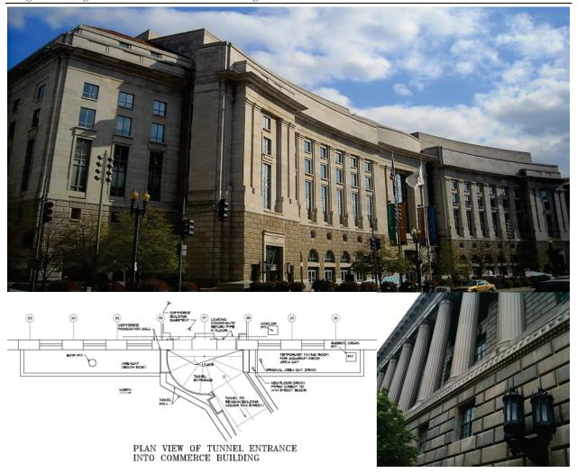
The scope of work was to determine the causes of the leaks and to propose remedies for repairing the leaks into the subject areas. The scope of work included an investigation of the leaking into the commerce tunnel that connected the Brand New Reagan Building with the 1900's Commerce Building. The work also included assessing the moisture that was infiltrating the basement slab from beneath as a result of an overwhelmed subsoil tile drain system.
