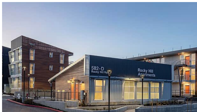
Rocky Hill Veterans' Housing - Vacaville, CA Energy Modeling, HERS Verification LEED-Gold Certification Support Program: CTCAC Certification: LEED-Homes Gold
