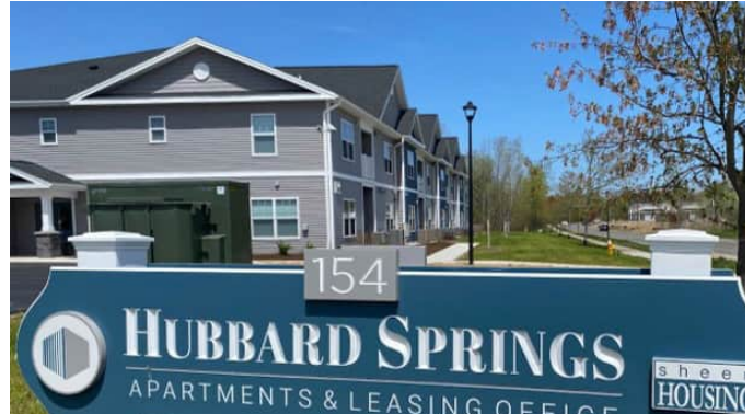
Hubbard Springs - North Chili, NY Energy Modeling, HERS Testing, LEED-Homes ENERGY STAR Homes Program: NY-HCR Certification: LEED-Homes
