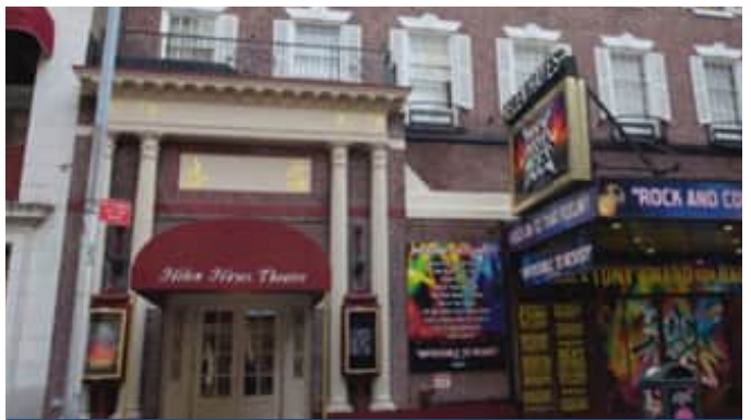
Helen Hayes Theater - New York, NY LEED Fundamental Commissioning LEED Enhanced Commissioning Certification: LEED Gold
