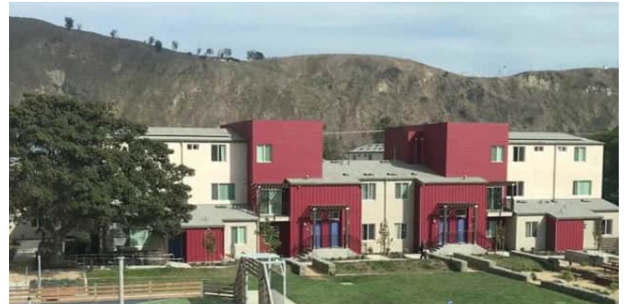
Westview Village - Ventura, CA Energy Modeling, Title 24 Compliance, CTCAC Application Support, CUAC Analysis, HERS Testing, LEED Certification Support Program: CTCAC Certification: LEED-ND, LEED-Homes
