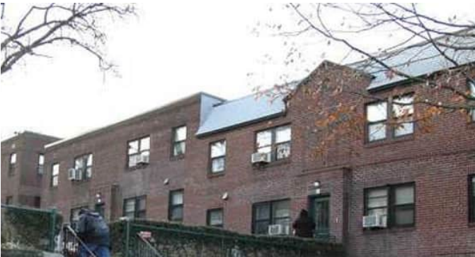
Awbury View - Philadelphia, PA Energy Modeling, EGC Certification Support, HERS Verification Program: PHFA Certification: Enterprise Green Communities
