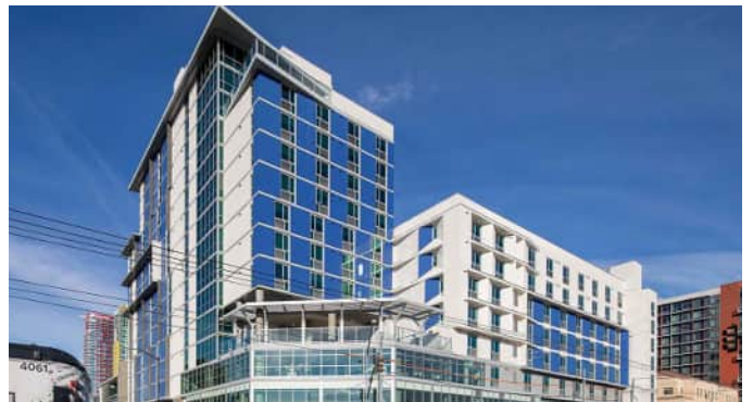
14th and Commercial Multifamily - San Diego, CA Title 24 Energy Modeling, HERS, CUAC Support LEED Fundamental Commissioning Program: CTCAC Certification: LEED-NC
