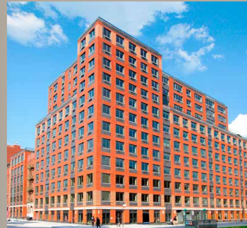
Above. The Balton, located in the heart of Harlem in New York City, NY, includes 156 apartment homes at different levels of affordability. This transit-oriented site, with major subway lines accessed across its entrance, includes a retail component comprising a Columbia University affiliate office, wine store, yoga studio and garage.
