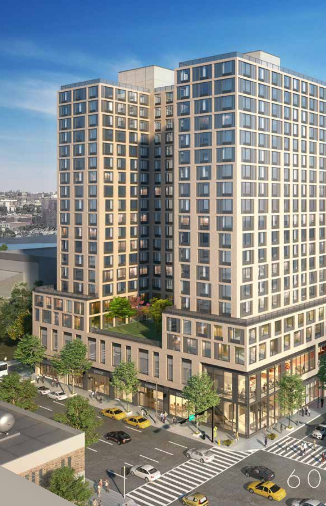
Left. 125th St B West is a mixed use, mixed income, transit-oriented site currently under construction in Harlem in New York City, NY. The site includes 404 apartment homes serving residents at different levels of affordability, from formerly homeless to market-rate units, over 60,000 square feet of retail and a 5,000-square-foot community facility.
