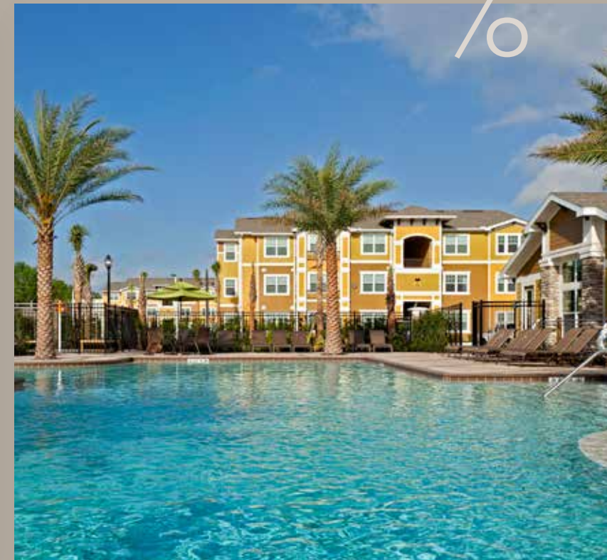
Bennett Creek, located in Jacksonville FL, includes 264 apartment homes, 60% market rate and 40% affordable.
