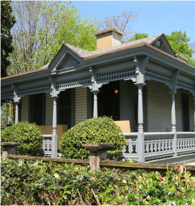
Figure 14. Image Illustrating Existing Neighborhood Architectural Character
