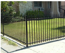
WROUGHT IRON METAL FENCE
