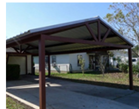
STEEL METAL FRAME CARPORT
