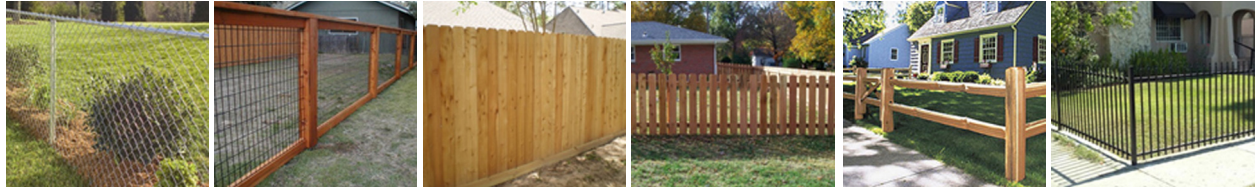
A - CHAIN LINK B - WOVEN METAL C - WOODEN SLAT D - WOOD PICKET E - RANCH STYLE F - WROUGHT IRON
