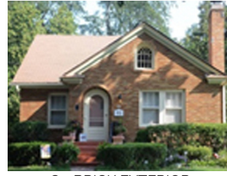
C - BRICK EXTERIOR
