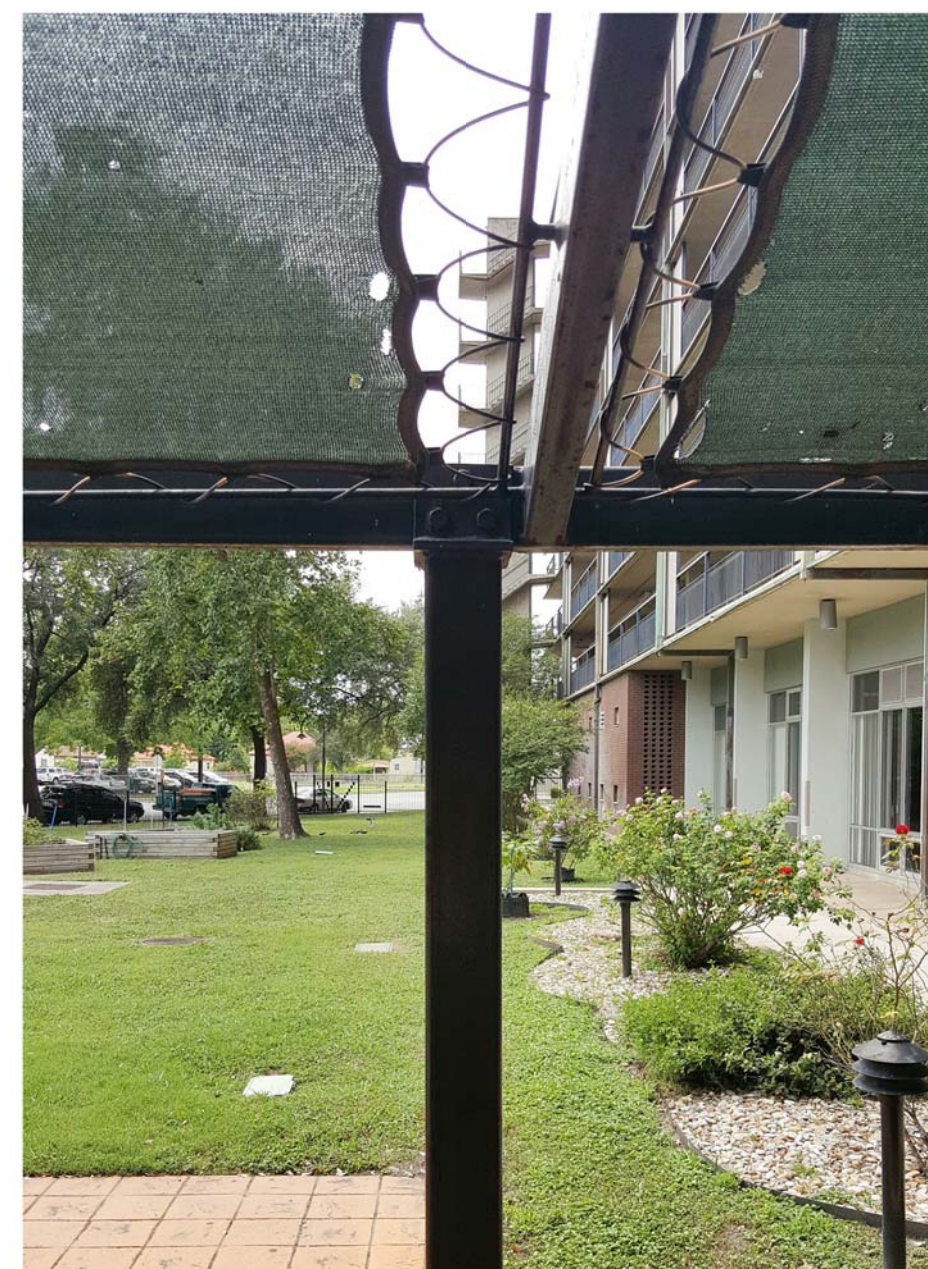
Existing canopy condition
