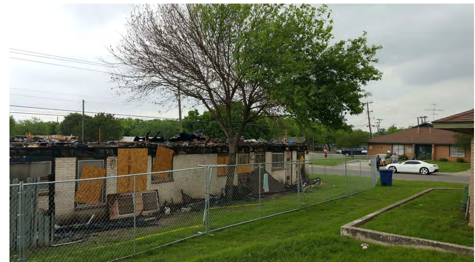
PHOTO II - EXISTING BUILDING REAR VIEW - N.T.S.
