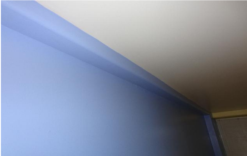
Photo #5 Pipe run bracket locations to be marked for installation by appropriate personnel.
