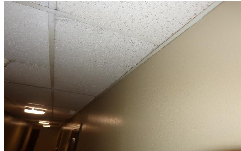
Photo #8 Pipe run bracket locations to be marked for installation by appropriate personnel.
