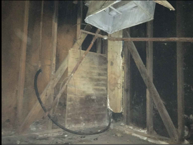
17: View of furnace hood and possible piping associated with the natural gas heating system.
