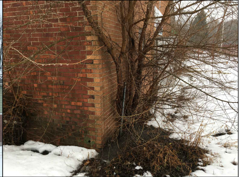
14: View of an unknown pipe sticking out of the ground and hole where piping may have been removed, on the northwest corner of the building.
