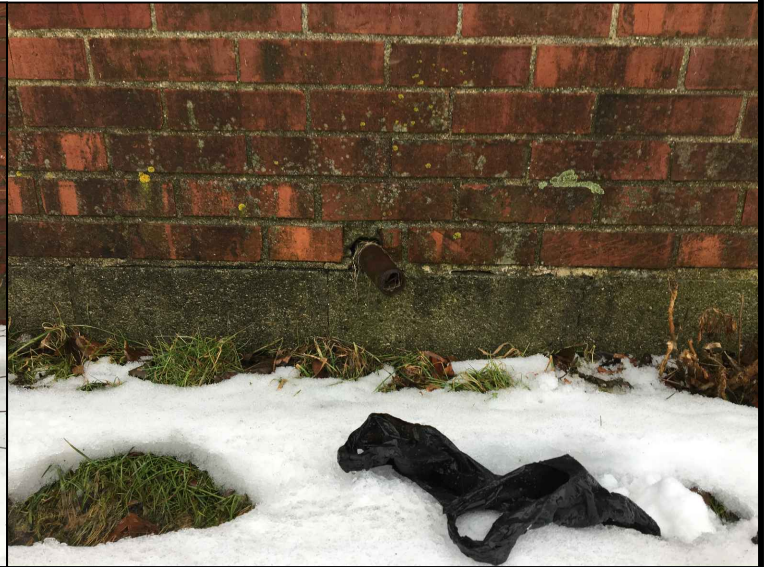
10: View of possible water drainage piping for baptistery located on the north side of the subject site building.
