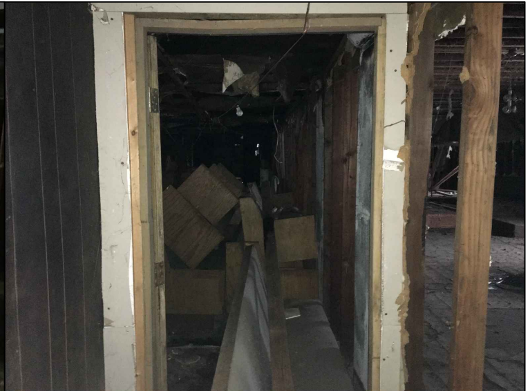
24: View of storage room area.
