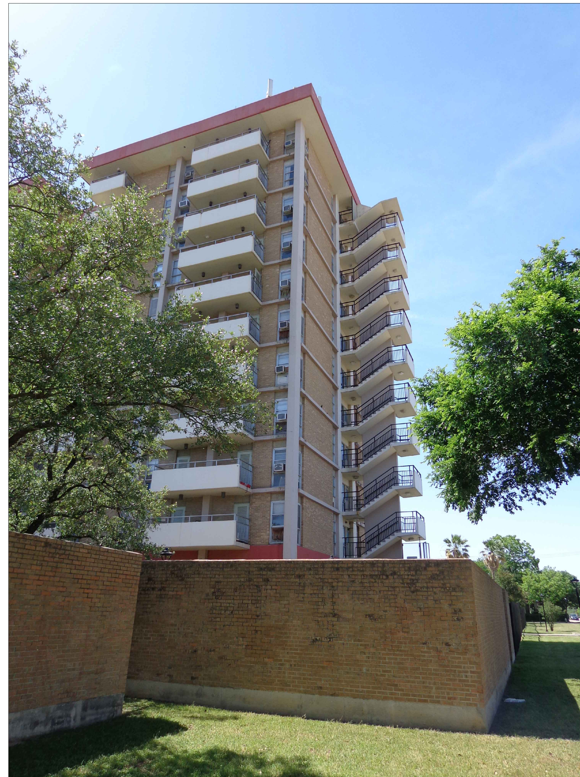
2 SOUTH ELEVATION PHOTO NTS
