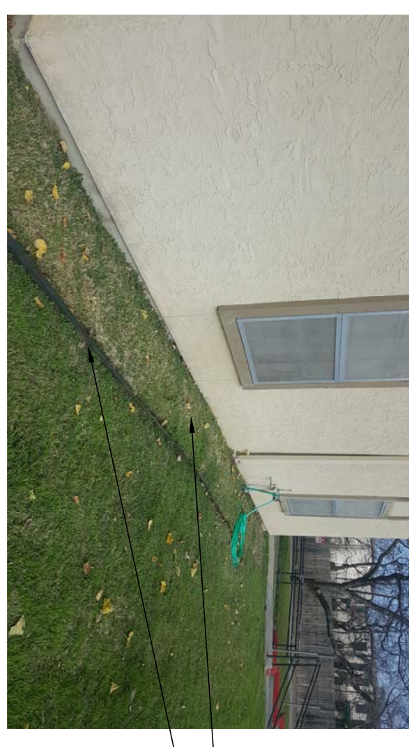
REGRADE THIS AREA TO DRAIN AS INDICATED LOWER GRADE AT ABANDONED PLANTER AND REMOVE ENTIRE METAL EDGER
