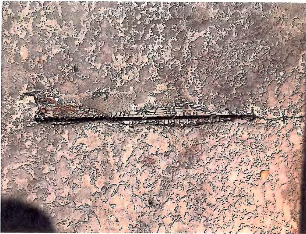
Photo 5 Cracks in coating
