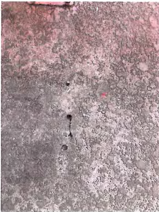
Photo 5 Cracks in coating
