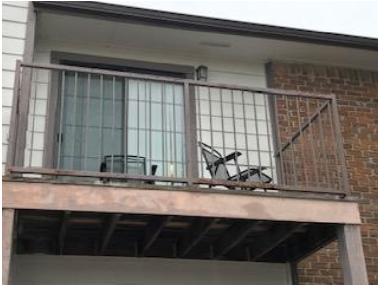
Typical balcony rails
