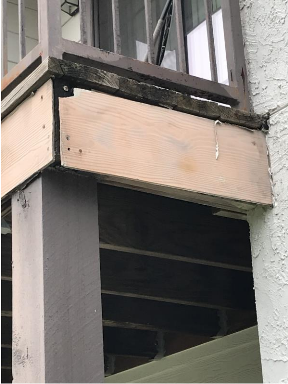
Typical repairs at balcony siding
