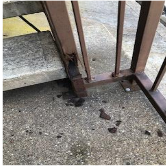
Stair column and girder
