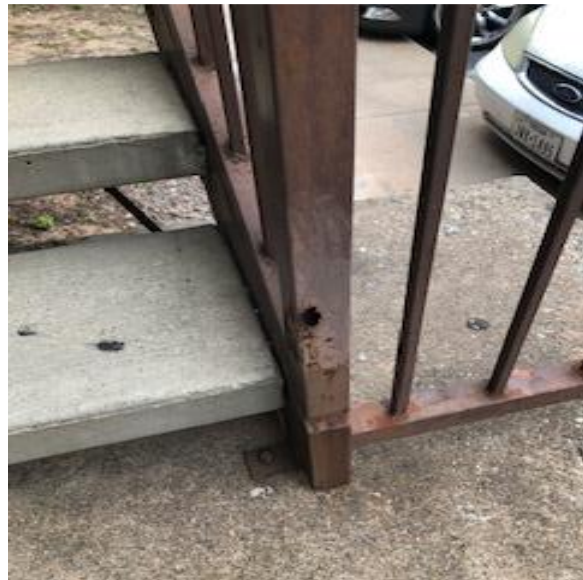
Stair tower post
