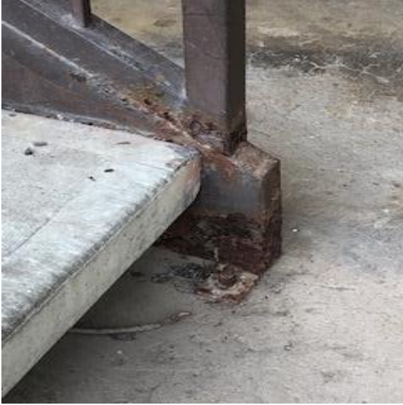
Stair post and girder
