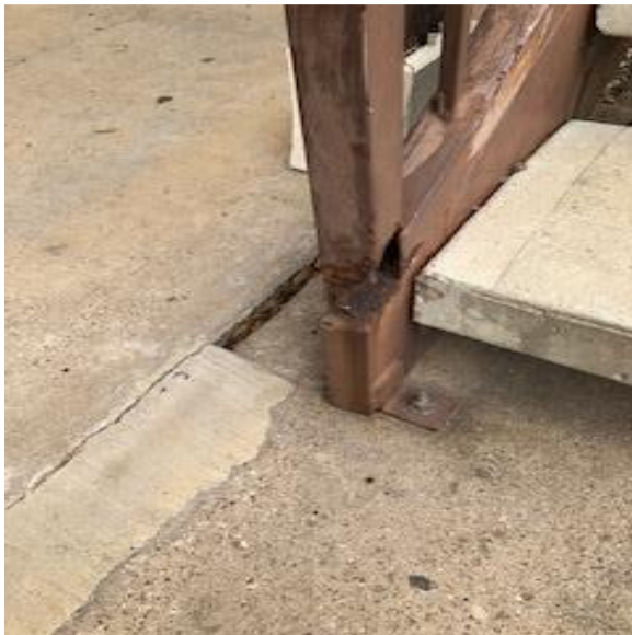
Stair post and stringer
