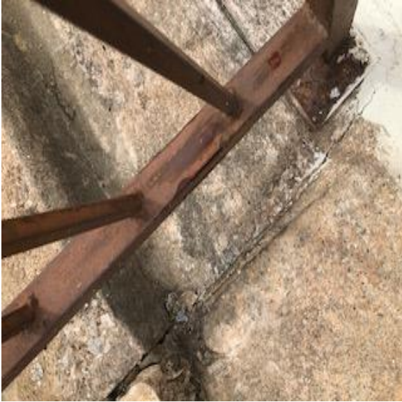
Bottom of step rail
