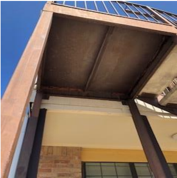
Typical condition under concrete landing at the stair towers
