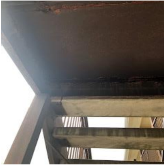
Under side of stair tower
