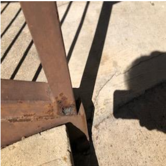
Stair tower post
