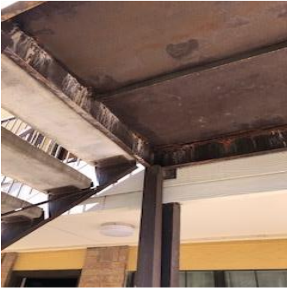
Typical rust under stair tower landing
