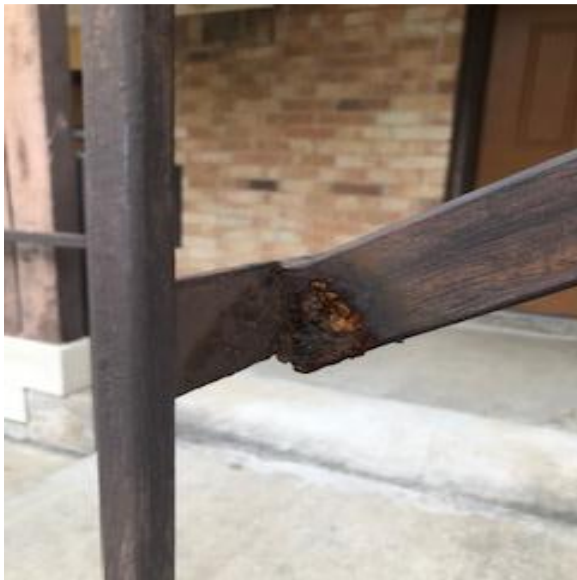
Handrail at stair tower
