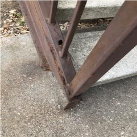
Stair post and stringer
