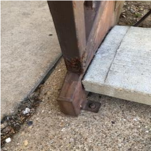
Stair post and girder
