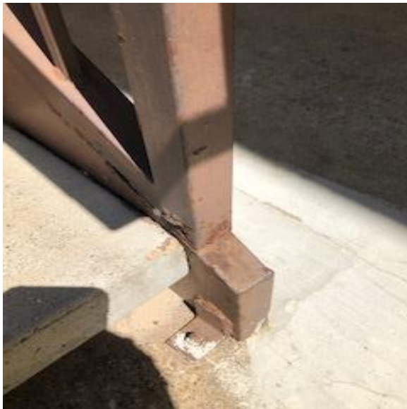
Stair post and girder
