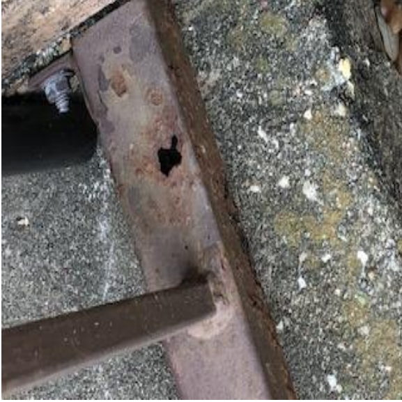
Bottom of rail
