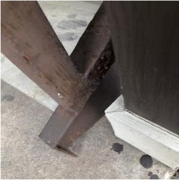
Stair post and stringer
