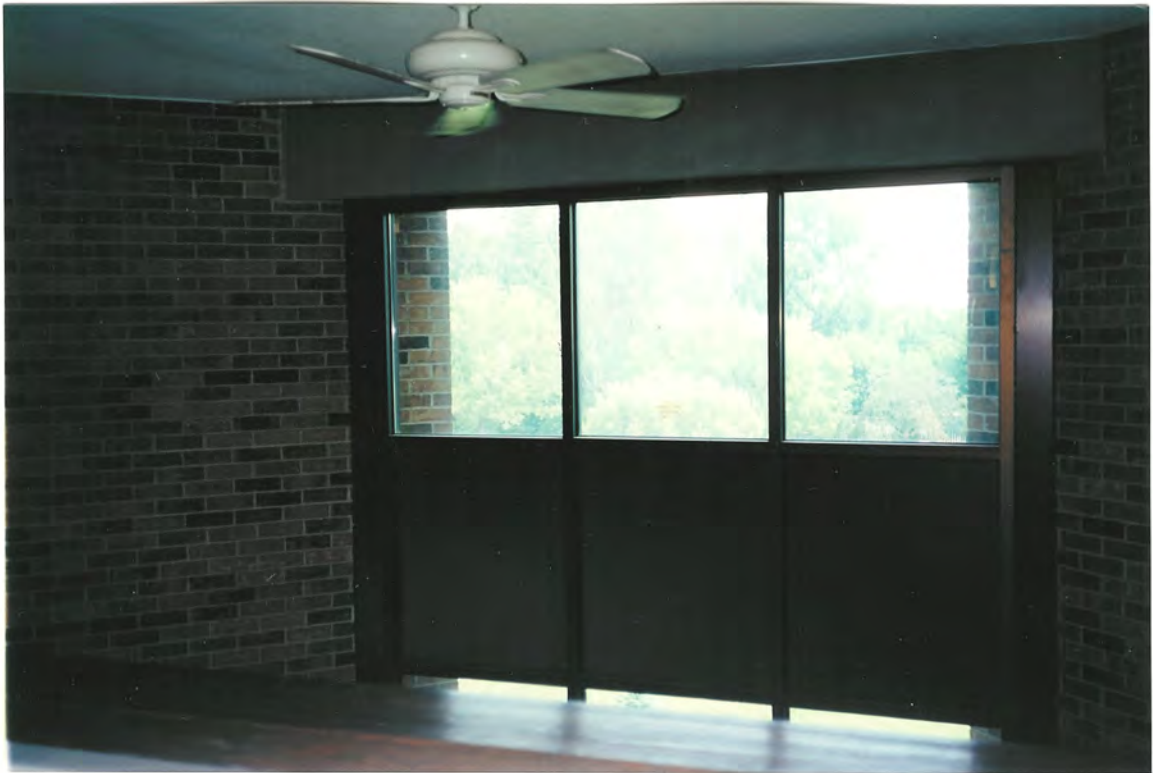
Plate 3: Showing exterior windows with black colored ACM Caulk.
