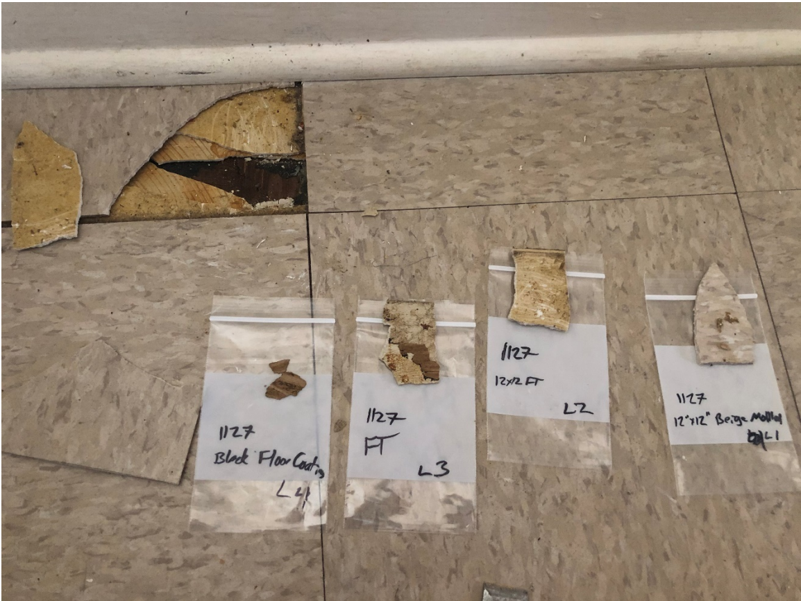
Photo 1: Multiple Layers of Flooring (typ.)
