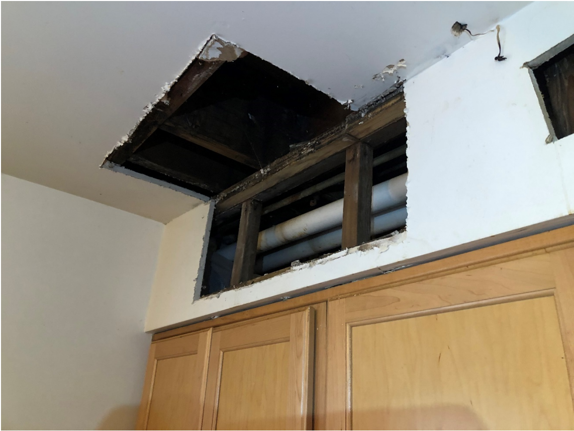
Photo 2: Drywall and Drywall Joint Compound
