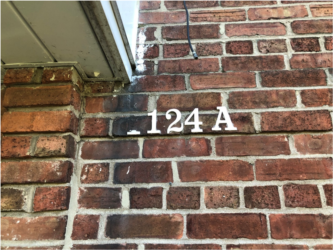
Photo 11: Exterior Brick and Mortar (typ.)
