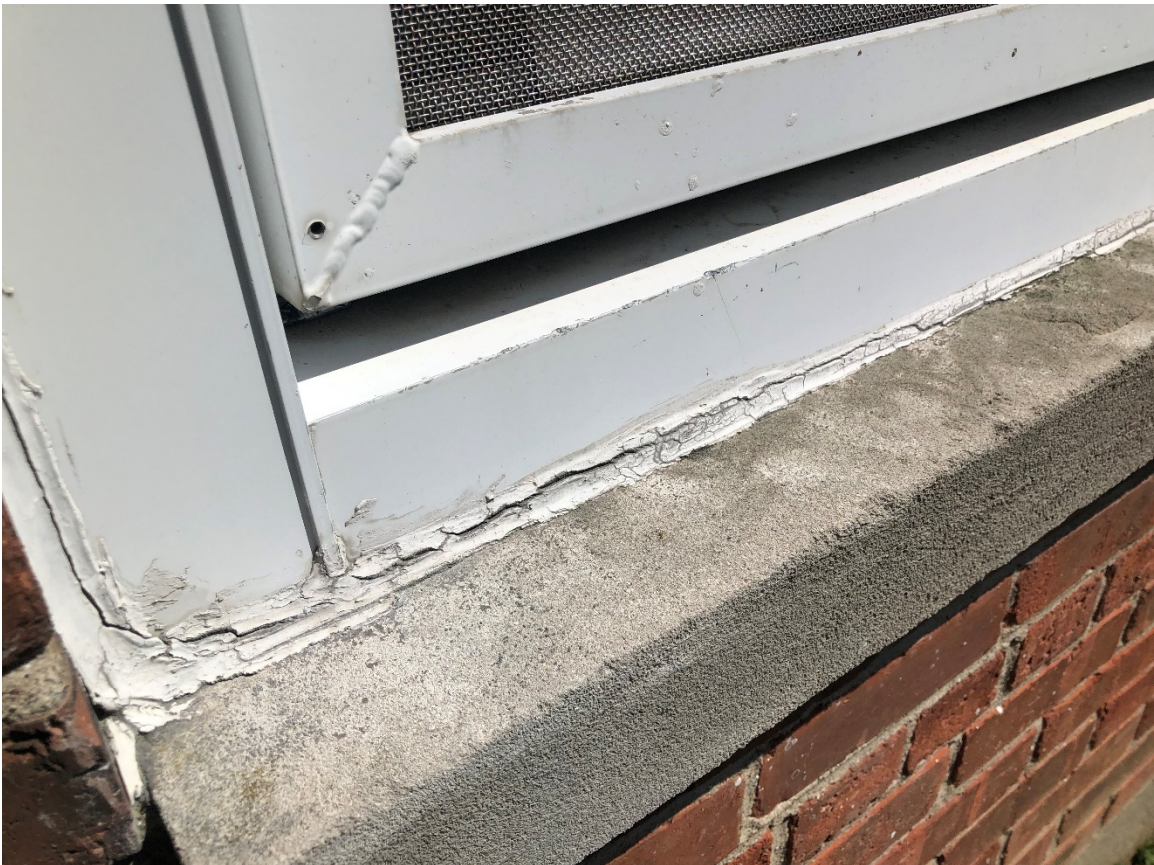
Photo 16: Exterior Window Caulk
