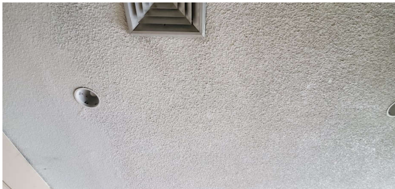
Photo 2: View of typical RACM popcorn ceiling finish.
