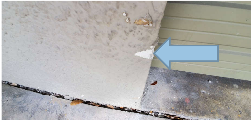
Photo 4: Typical ACM stucco sampled during this inspection.
