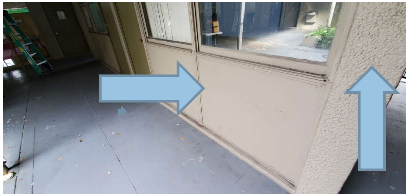
Photo 5: ACM Transite panels and exterior stucco identified during this inspection.
