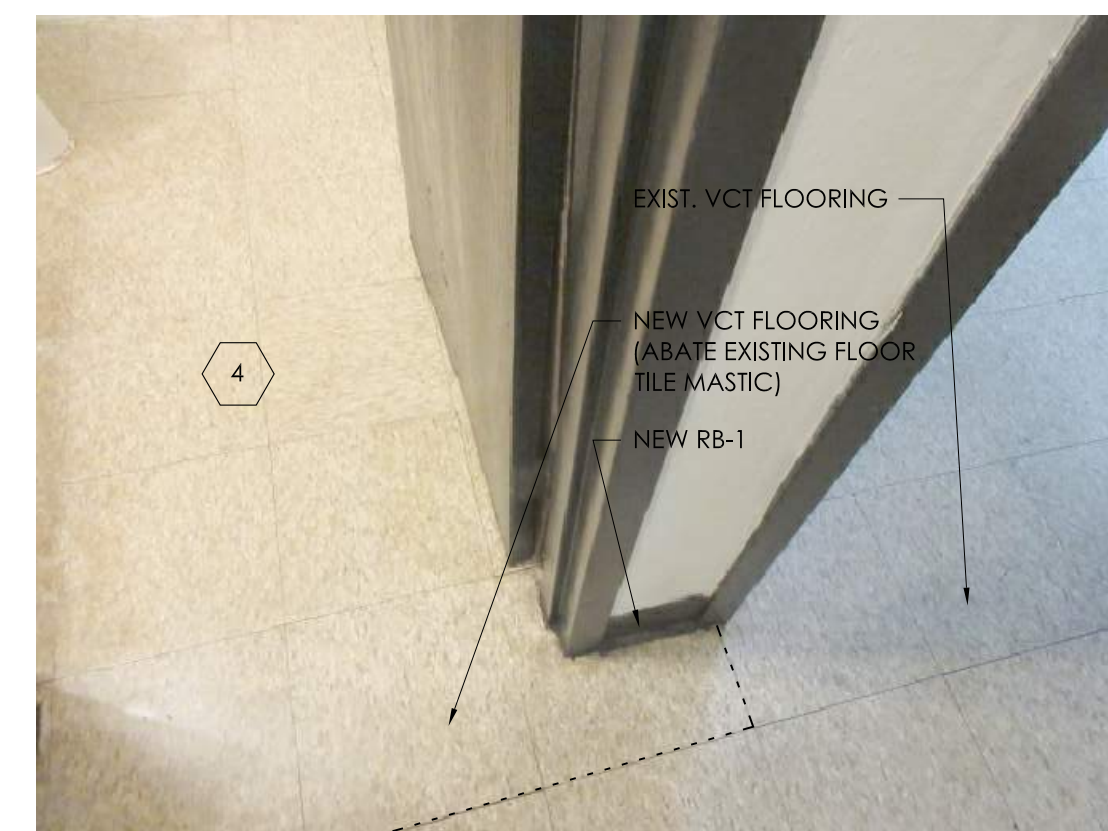
8 EXISTING BATHROOM PHOTO A3.0 NOT TO SCALE
