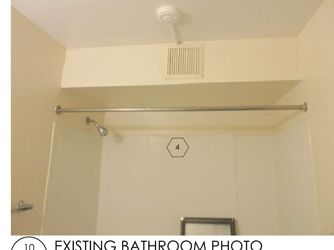
10 EXISTING BATHROOM PHOTO A3.0 NOT TO SCALE
