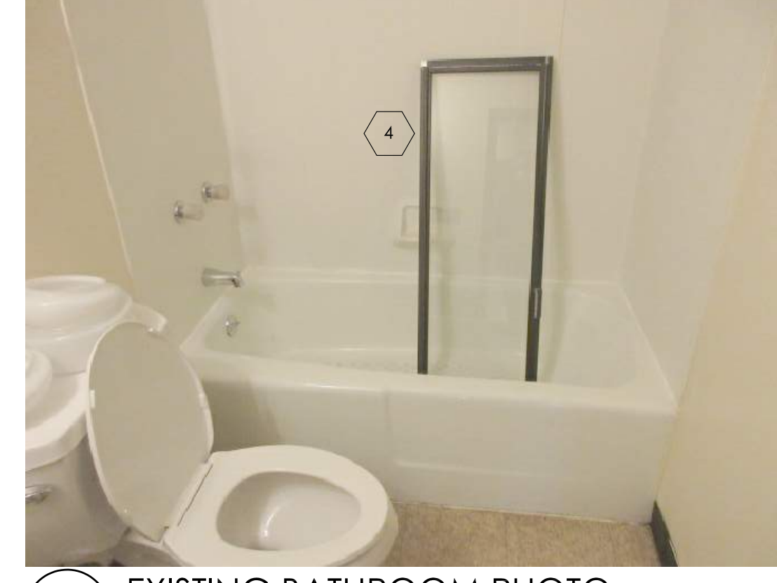
9 EXISTING BATHROOM PHOTO A3.0 NOT TO SCALE
