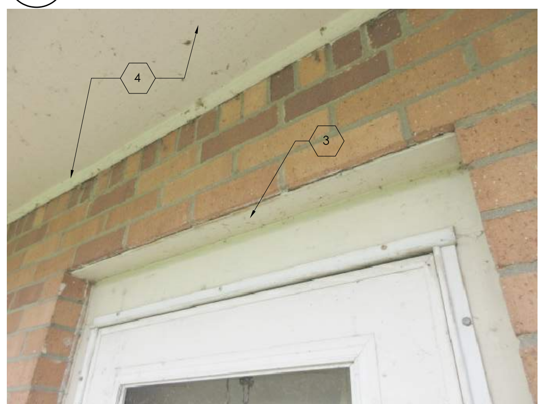
2 TYPICAL LINTEL @ DOOR A2.0 NOT TO SCALE
