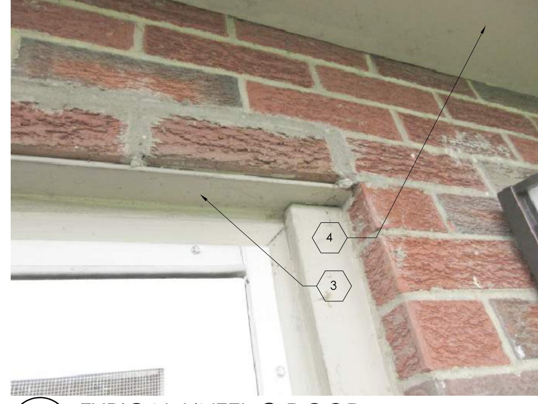
7 TYPICAL LINTEL @ DOOR A2.0 NOT TO SCALE
