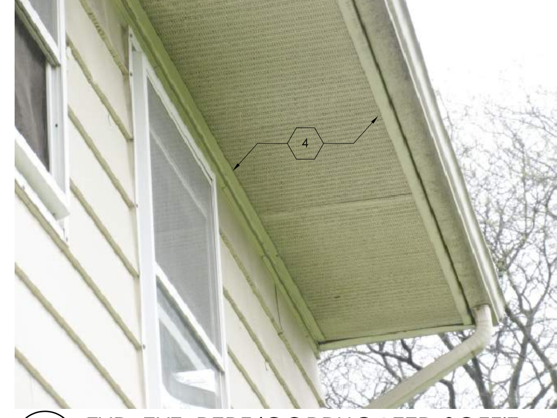
10 TYP. EXT. PERF/CORRUGATED SOFFIT A2.0 NOT TO SCALE
