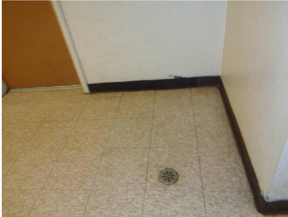
Photo 7: Typical view of brown cove base (BCA, non-asbestos) found throughout the facility common areas.
