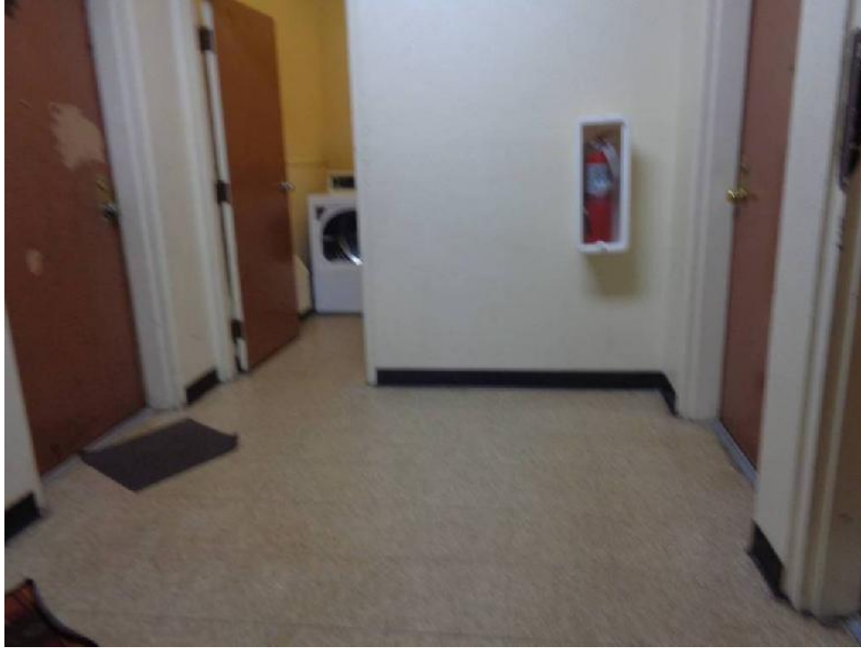
Photo 21: View of beige floor tile (FTA, non-asbestos) from the second floor hallway and laundry room of 9845 Oak Place Court common area.
