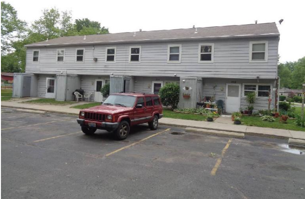
Photo 2: General view of the facility exterior.
