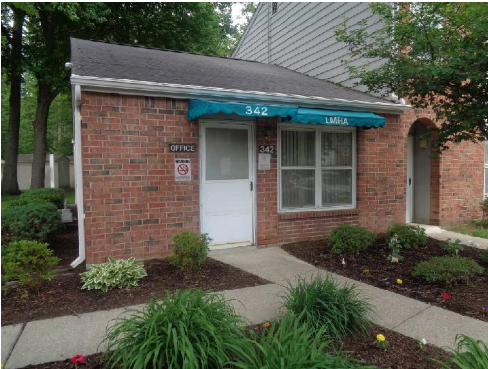
Photo 10: View of Oak View Court office building.
