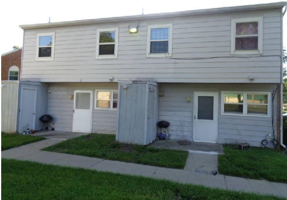
Photo 3: General view of the facility exterior.
