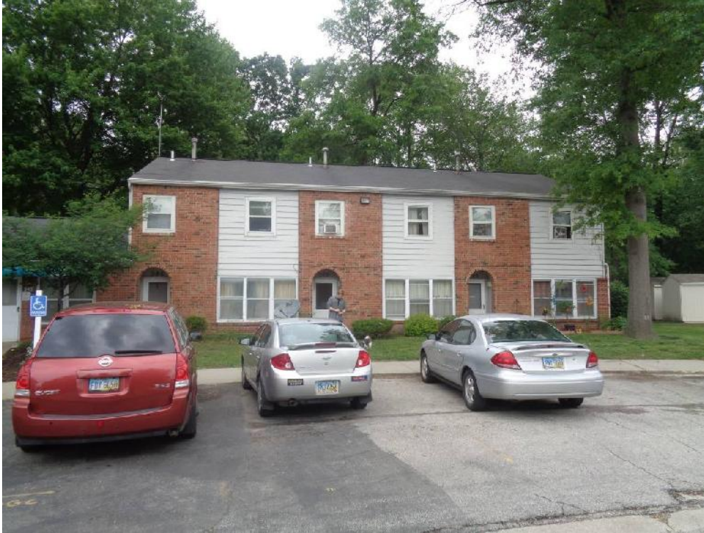
Photo 1: General view of the facility exterior.
