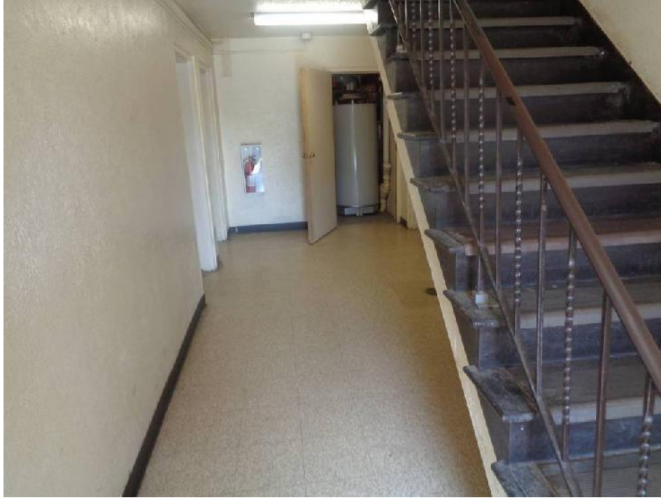
Photo 19: View of beige floor tile (FTA, mastic is asbestos containing), brown stair tread (STA, non-asbestos), drywall (DWA, non-asbestos), and black cove base (BCA, non-asbestos) from the common areas of 9842 Oak Place Court.
