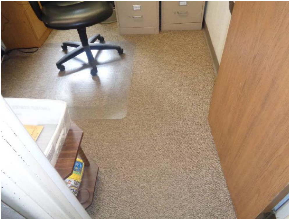
Photo 12: View of carpet and gray cove base (CBA, non-asbestos) in office building.
