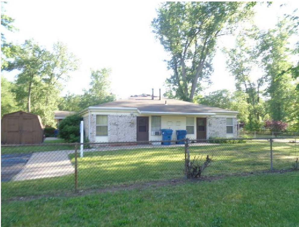
Photo 4: General view of the facility exterior.
