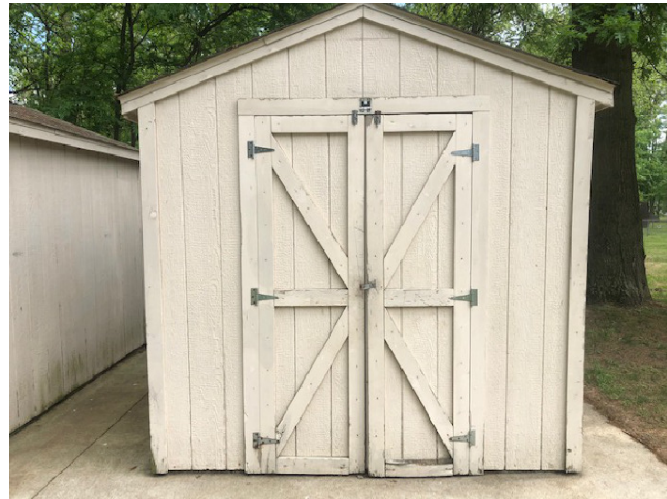
TYPICAL FRONT OF DETACHED STORAGE UNITS. NOTE LIMIT TO MOVING DOORS APART AND INCREASING WIDTH OF DOORS.
