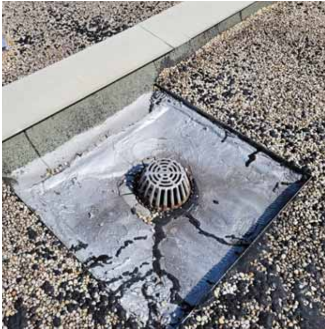
Photo 21: View of typical roof drain style
