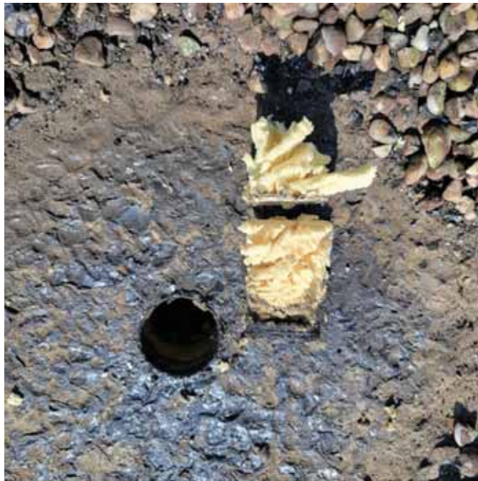
Photo 18: View of the Roof Core
