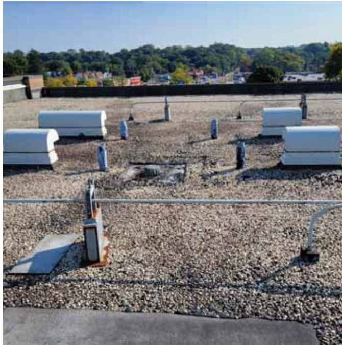
Photo 3: View of the Roof Field/Core (C-1,2,3,4)
