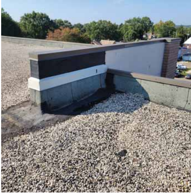
Photo 11: View of the Roof Flashing
