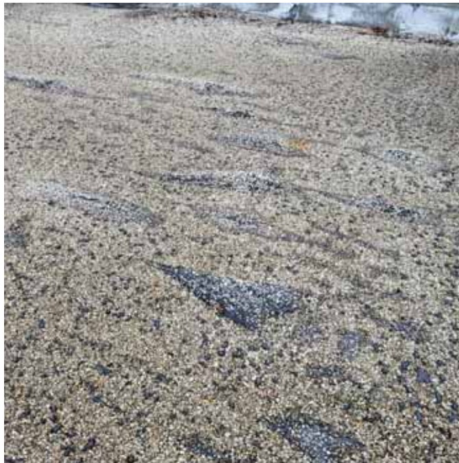
Photo 24: View of the Roof Field/Core
