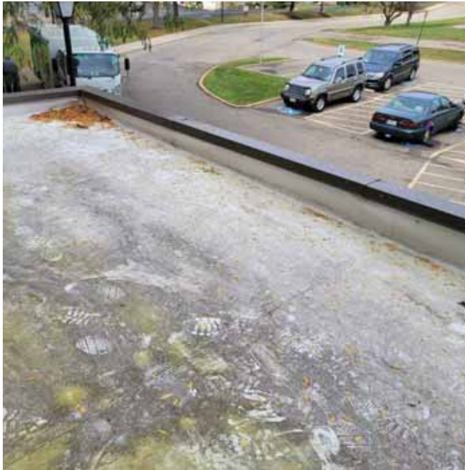
Photo 29: View of the lower Roof Field/Core (C-6,7)
