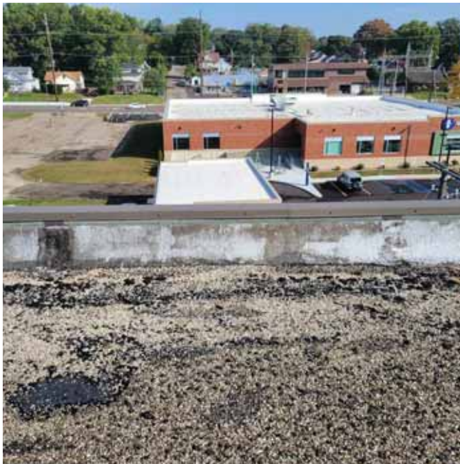
Photo 6: View of the Roof Flashing
