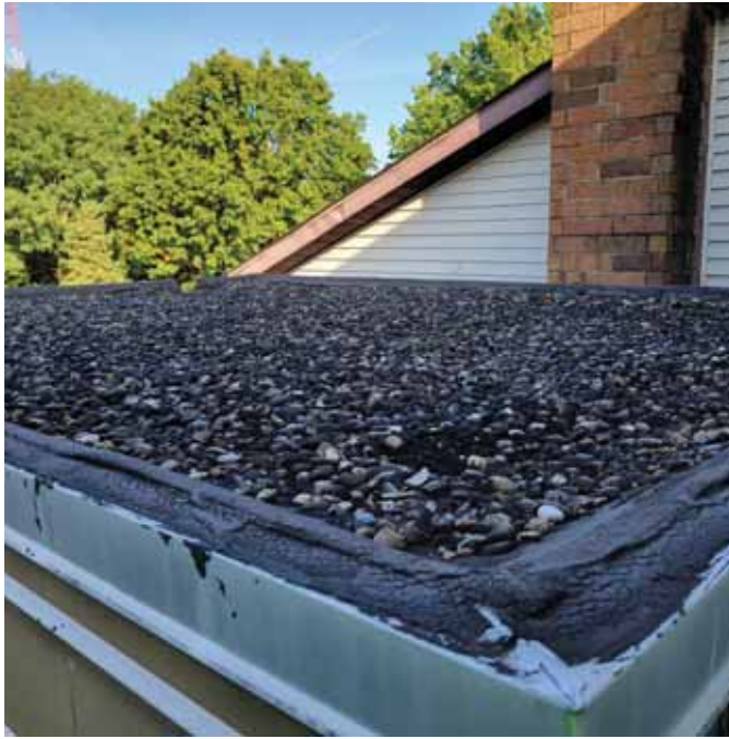
Photo 5: View of the upper flat roofing area
