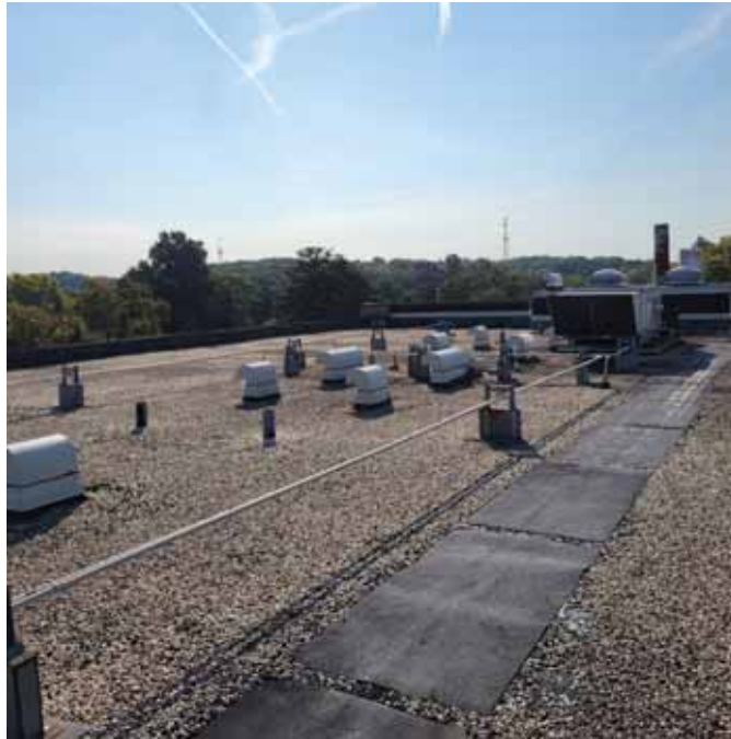
Photo 5: View of the roof looking South
