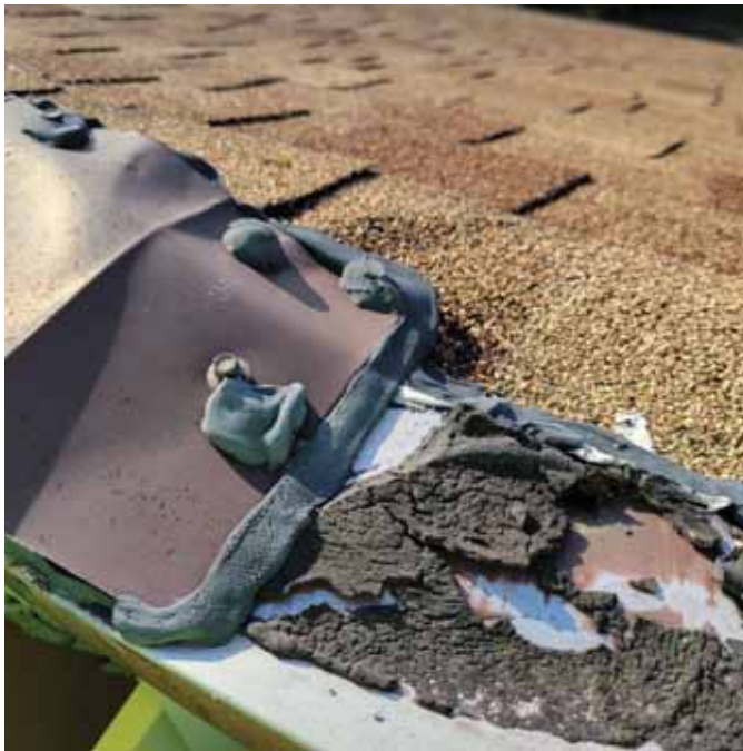
Photo 10: View of the upper shingled roofing areas and tar
