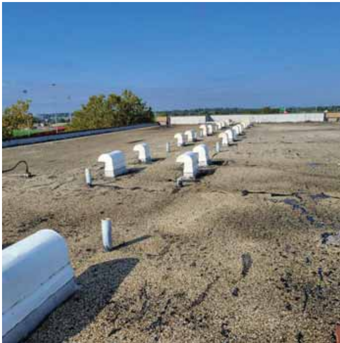
Photo 12: View of the West portion of the roof
