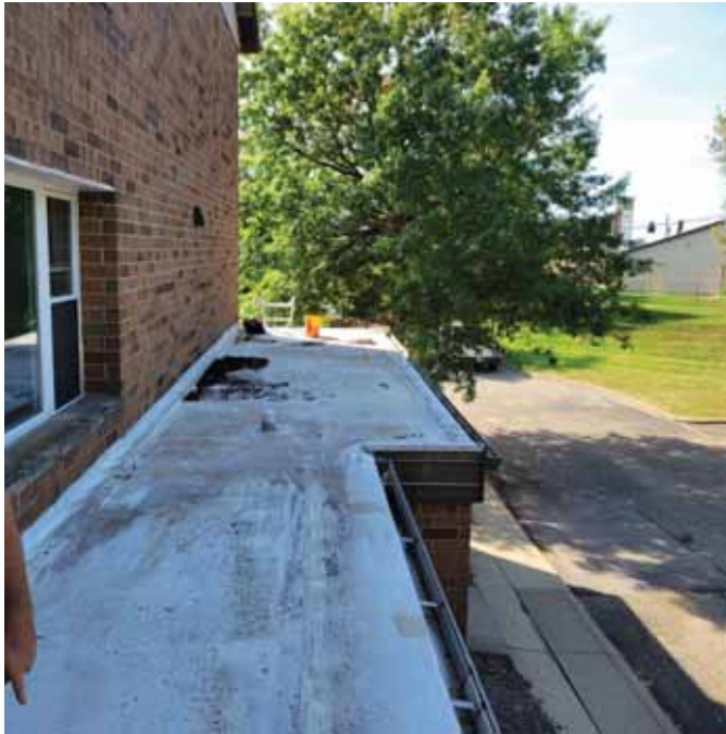
Photo 18: View of the lower roof areas
