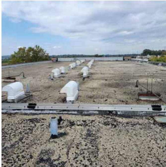
Photo 27: View of the West portion of the roof
