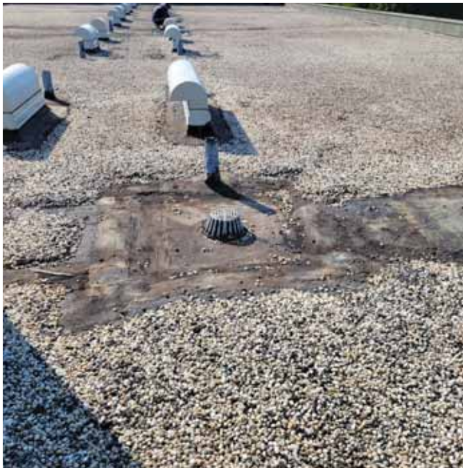
Photo 10: View of recent patching on the roof
