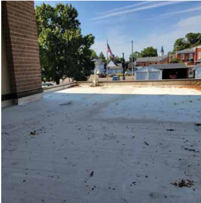
Photo 23: View of the lower roof near the front entrance
