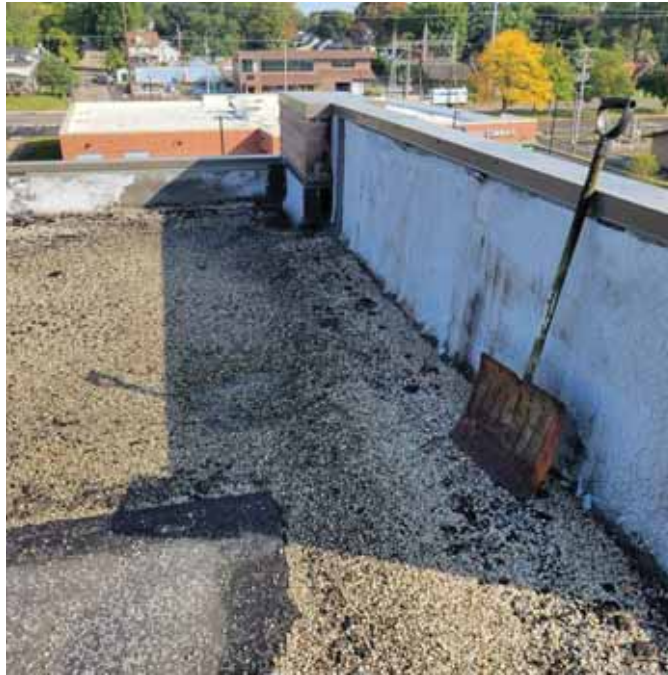
Photo 1: View of the Roof Flashing (F-1,2)
