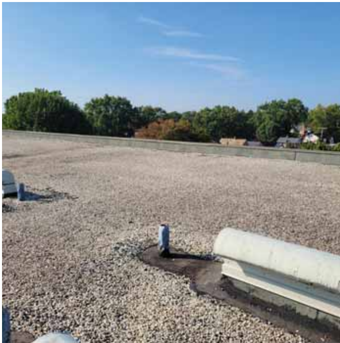
Photo 14: View of the southern portion of the roof
