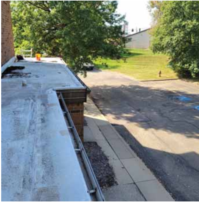
Photo 17: View of the lower roof areas
