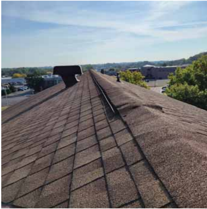
Photo 7: View of the upper shingled roofing areas
