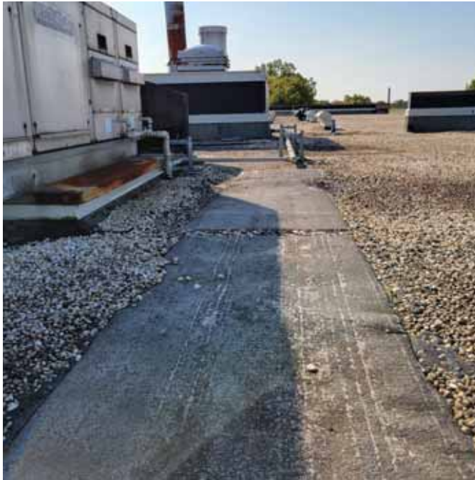
Photo 9: View of the walkway warping and bubbling
