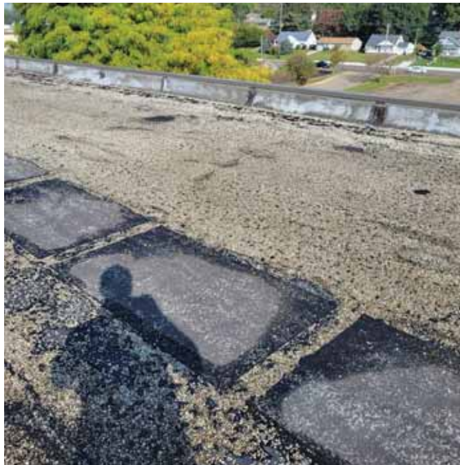
Photo 2: View of the Roof Field/Core (C-1,2,3,4)
