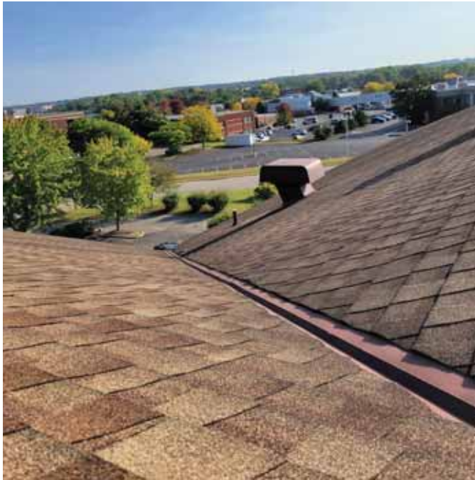
Photo 8: View of the upper shingled roofing areas
