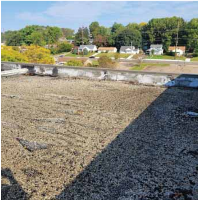
Photo 9: View of the Roof Flashing North
