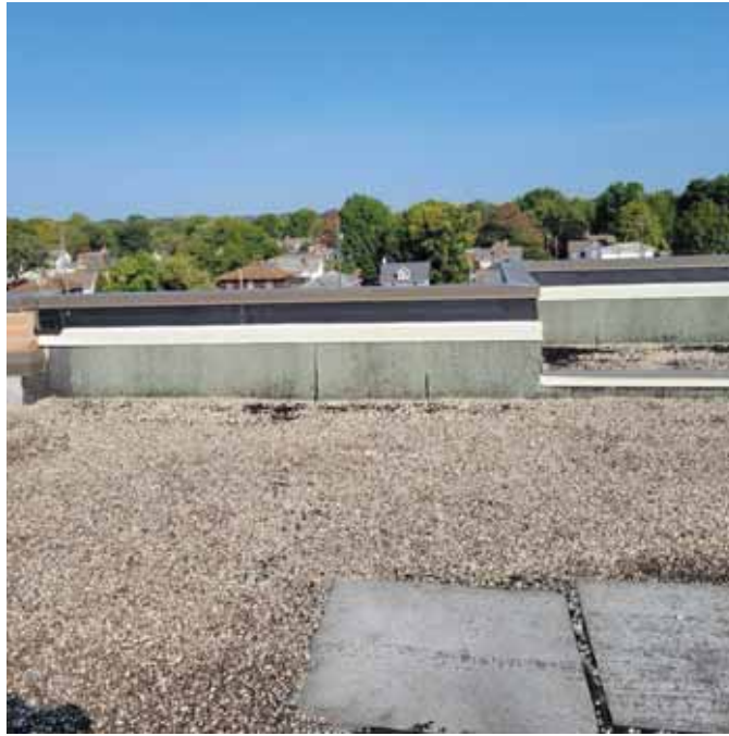
Photo 1: View of the Roof Flashing (F-1,2)
