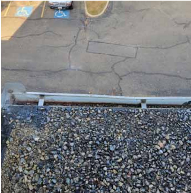
Photo 3: View of the upper flat roofing area Field/Core
