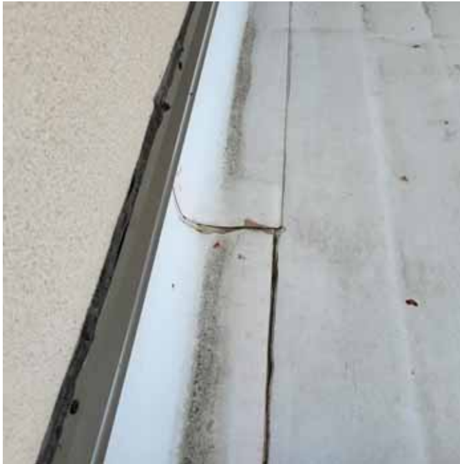
Photo 24: View of the lower roof flashing (F-3,4) near the front entrance
