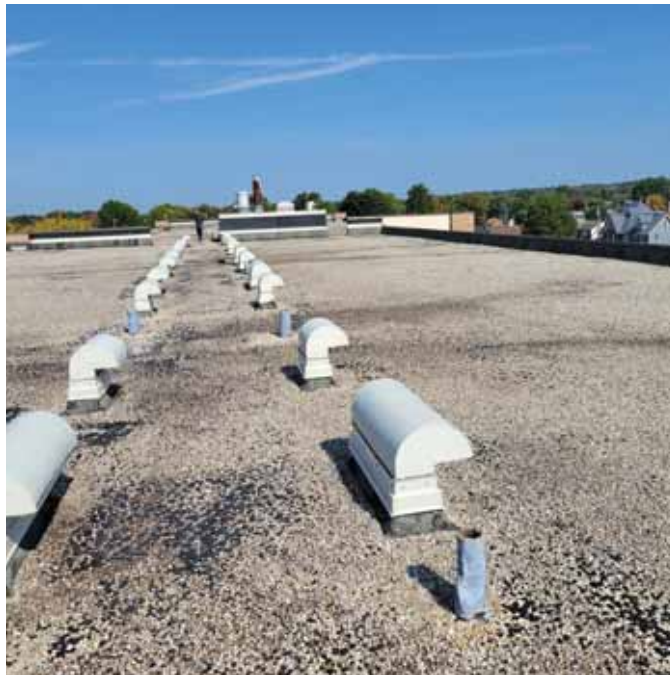
Photo 20: View of the Roof looking North
