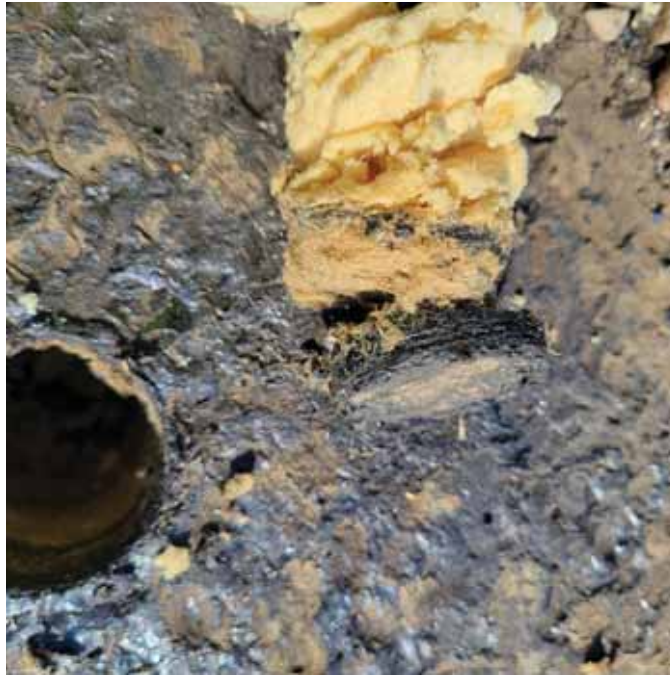
Photo 19: View of the Roof Core layers
