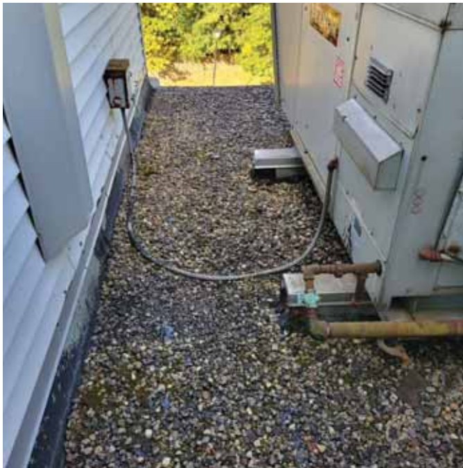
Photo 4: View of the upper flat roofing area
