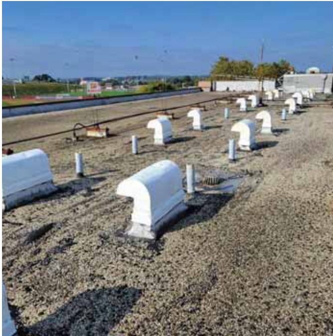
Photo 3: View of the Roof Field/Core (C-1,2,3,4) looking West
