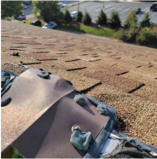
Photo 9: View of the upper shingled roofing areas and tar(C-3,4)
