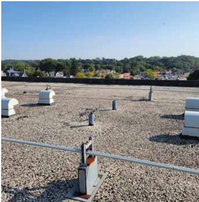
Photo 8: View of the Roof Field/Core
