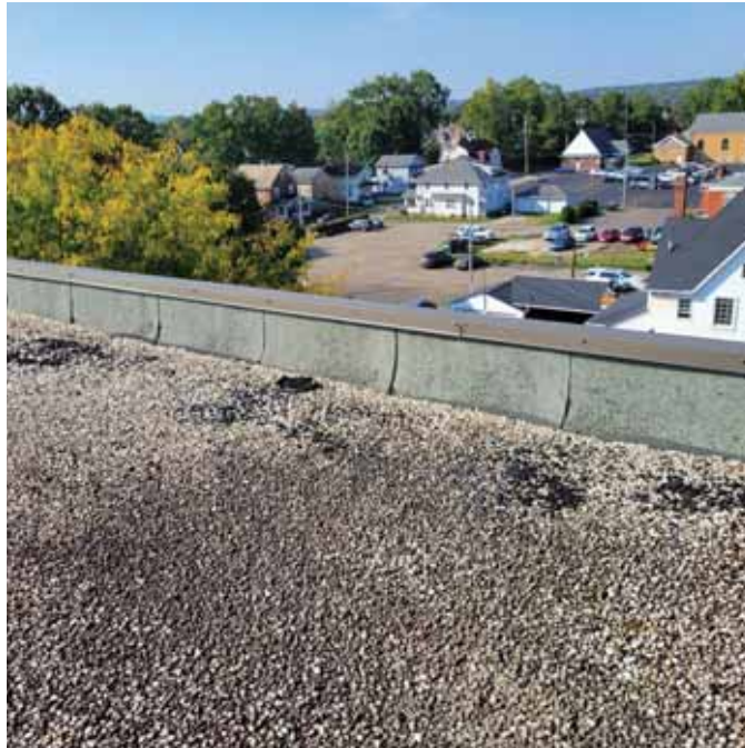
Photo 2: View of the Roof Flashing
