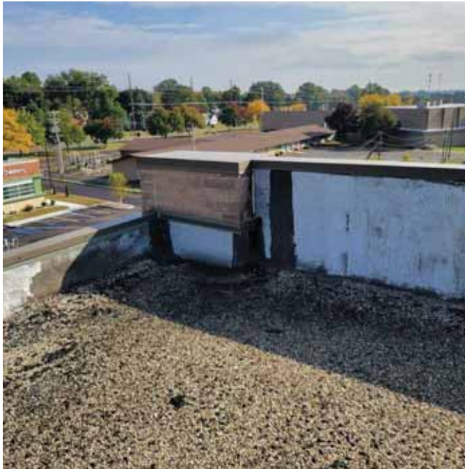
Photo 5: View of the Roof Flashing
