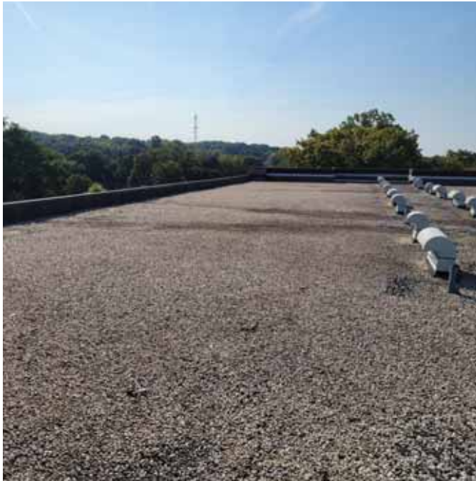
Photo 13: View of the southern portion of the roof
