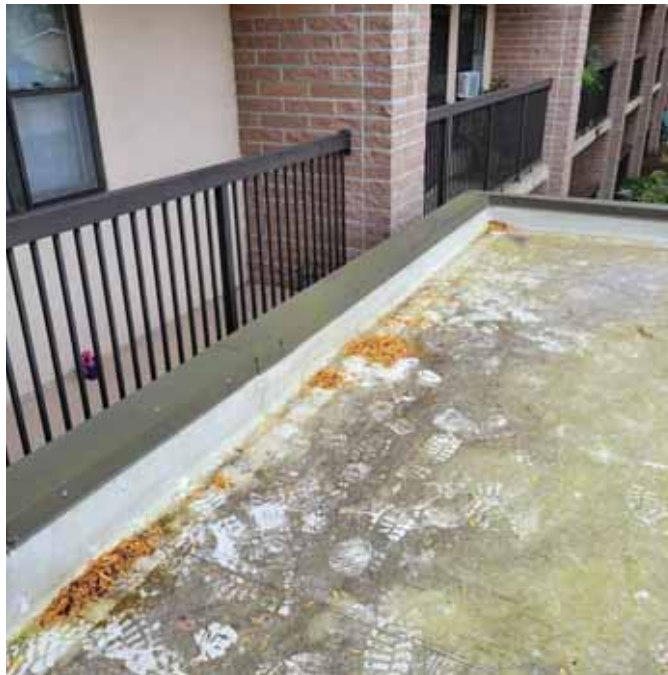
Photo 28: View of the lower roof Flashings (F-3,4)
