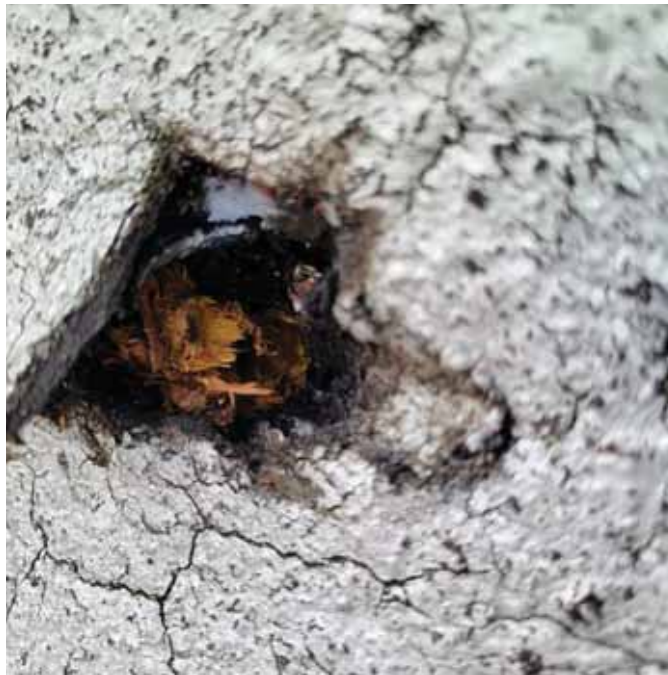
Photo 22: View of flashing to substrate
