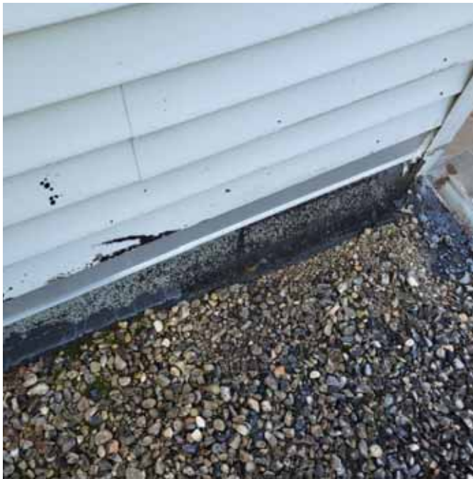
Photo 2: View of the upper flat roofing area Roof Flashing (F-1,2)
