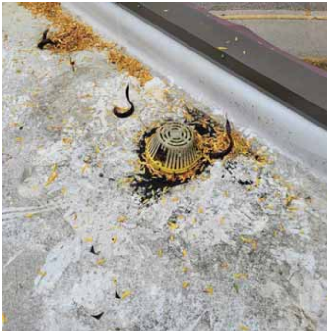
Photo 30: View of typical roof drain on the lower roof
