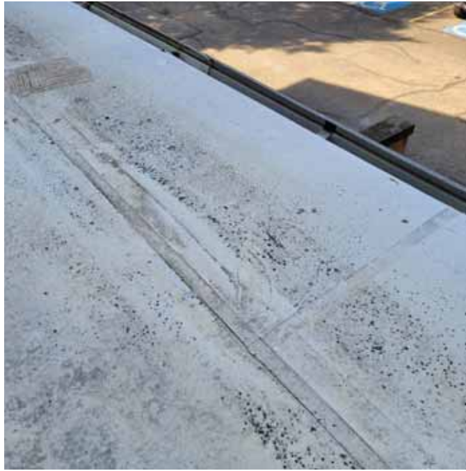
Photo 13: View of the lower roof areas (C-5,6)
