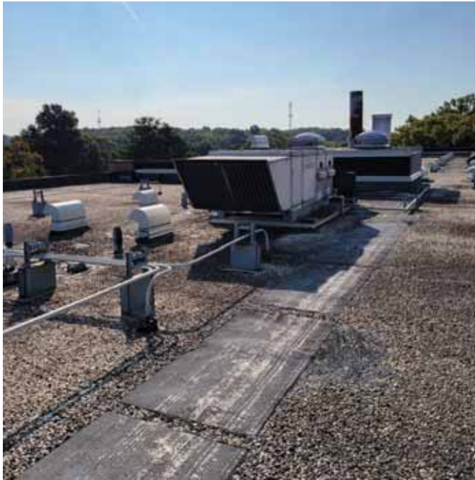
Photo 7: View of the Rooftop Units and Walkway
