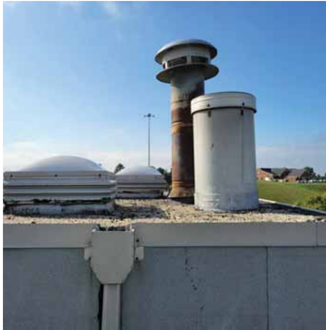
Photo 21: View of the elevator penthouse
