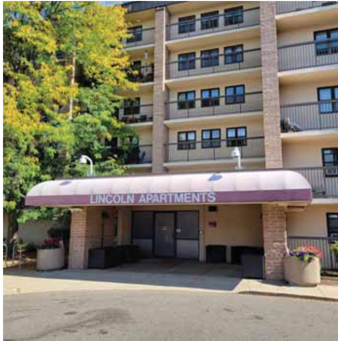
Photo 25: View of the main entrance to the property
