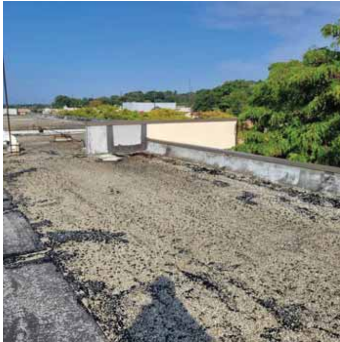
Photo 8: View of the North parapet wall
