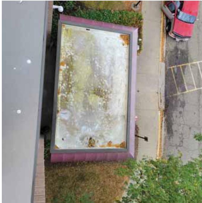
Photo 23: View of the lower roof from the upper roof
