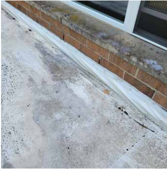
Photo 19: View of the lower roof areas
