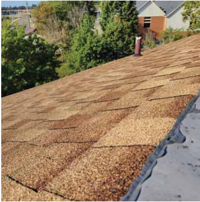
Photo 11: View of the upper shingled roofing areas
