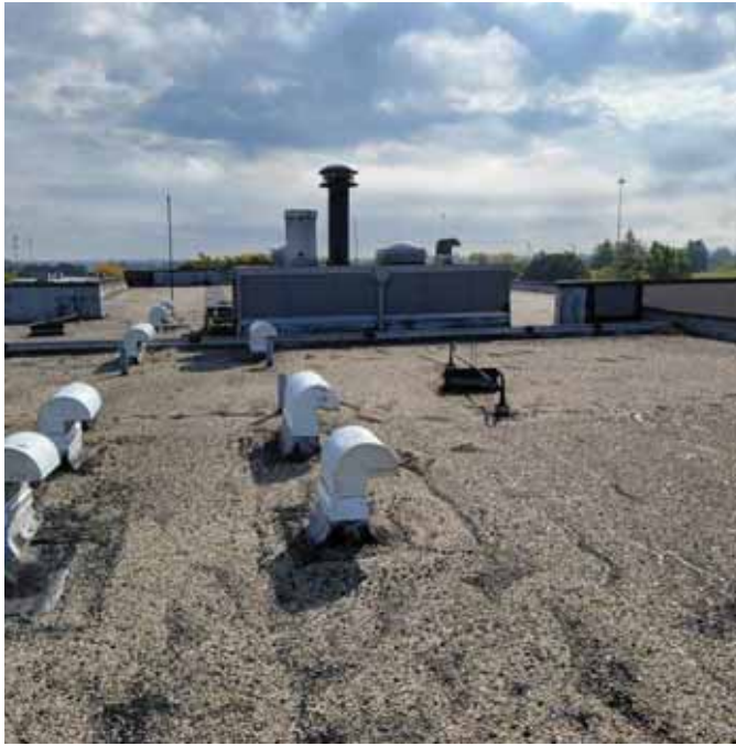
Photo 19: View of the elevator penthouse (C-5)
