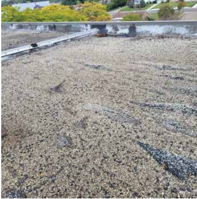
Photo 25: View of the Roof Field/Core
