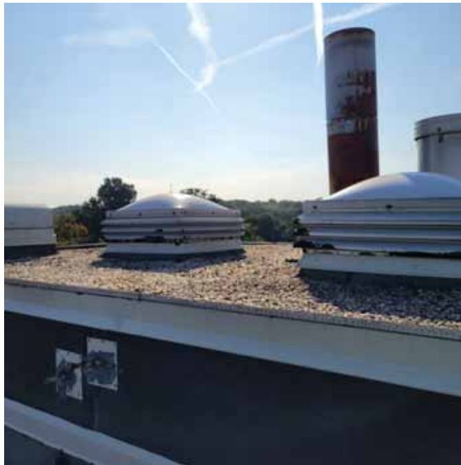
Photo 4: View of the elevator penthouse (C-5 location)
