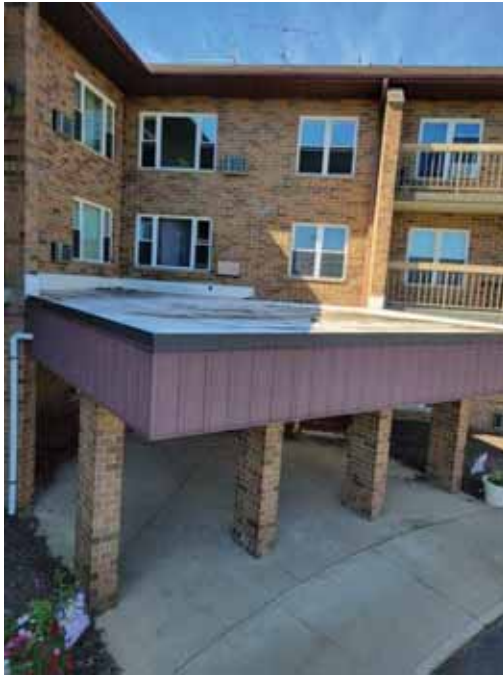
Photo 21: View of the front entrance roof flashings (F-5,6) and field/core (C-7,8)
