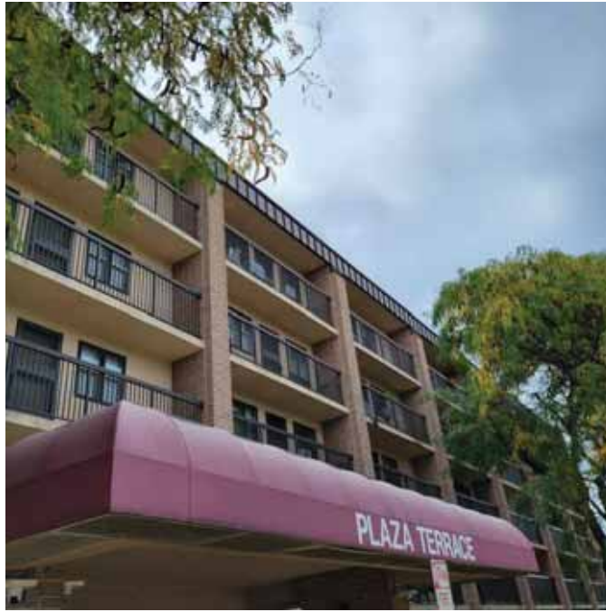
Photo 31: View of the main entrance to the property
