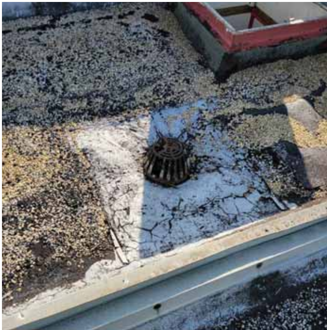
Photo 4: View of the typical drain system of the roof
