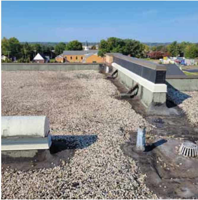
Photo 15: View of the western parapet wall
