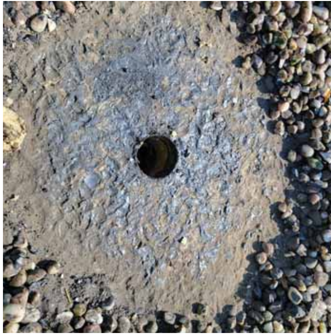
Photo 17: View of the Roof Core
