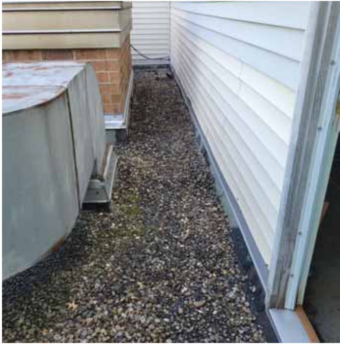
Photo 1: View of the upper flat roofing area (C-1, 2)
