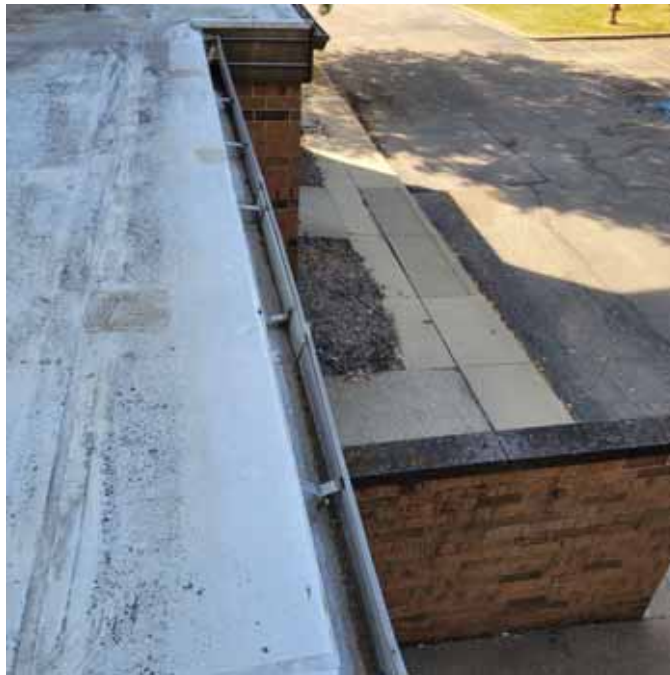
Photo 16: View of the lower roof areas
