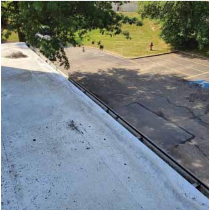
Photo 20: View of the lower roof areas
