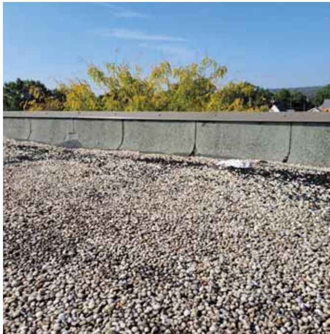
Photo 6: View of the Roof Flashing
