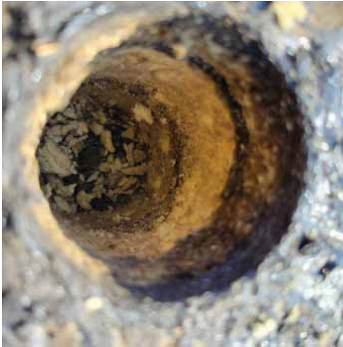
Photo 16: View of the Roof Core
