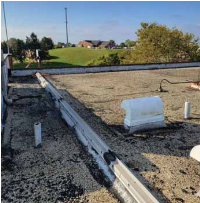
Photo 10: View of the Roof Flashing South
