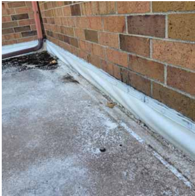
Photo 14: View of the lower roof flashings (F-3,4)
