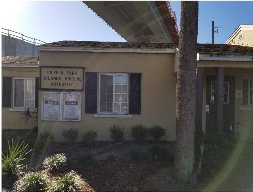
XRF-1 Exterior Office Building Side A Yellow Paint on Stucco (NLC)
