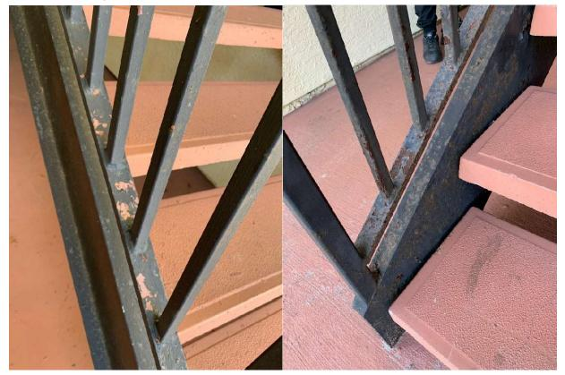
Open ends on the railings shall be enclosed (such as welding on a metal cap) to prevent air and moisture from getting inside the railings and causing the oxidation process to accelerate. Damaged kickplates, such as seen below on the right, shall be replaced prior to the application of the new paint schedule. There are eight (8) missing endcaps; contractor to verify quantity.
