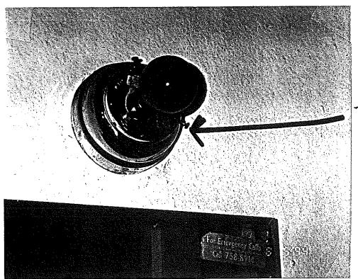
TYPICAL WALL LIGHT FIXTURE ANE ASSUMED TO CONTAIN ACM WIRING
