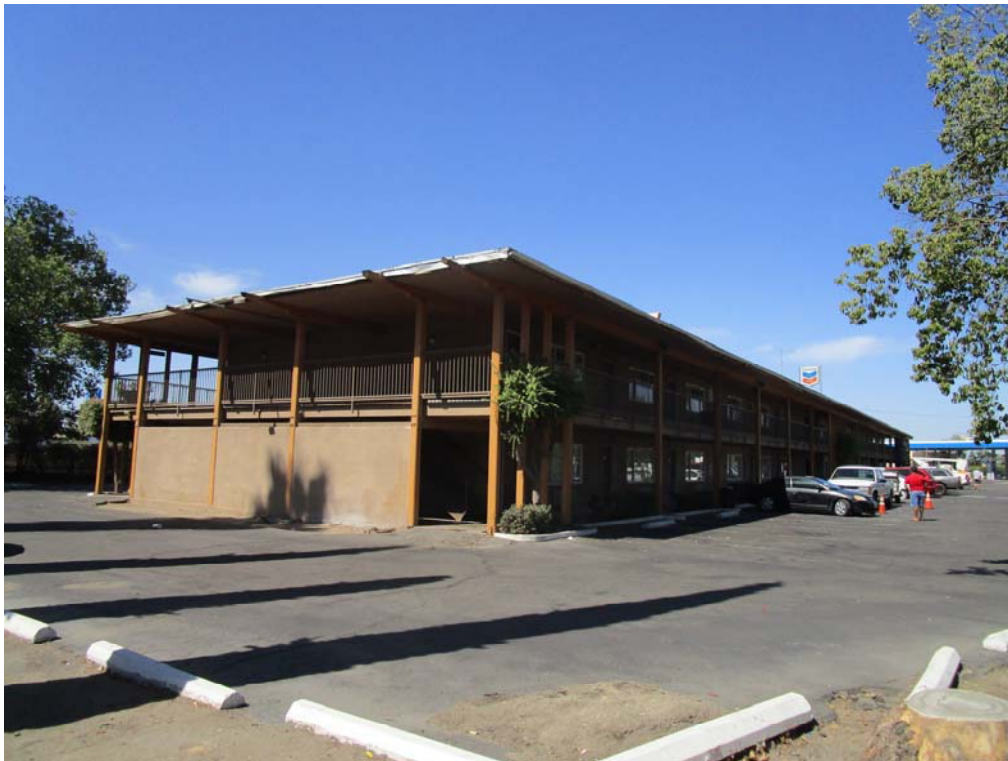
Photo 2: Southern center portion of subject site, facing north. Two-story motel building in foreground.
