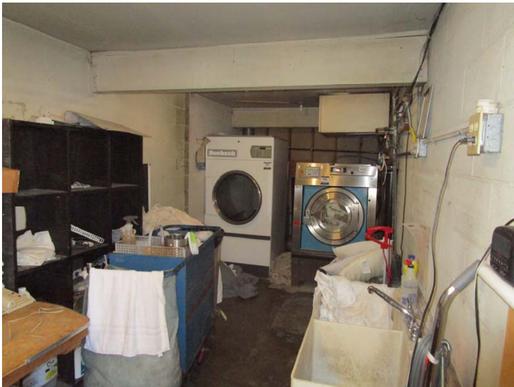
Photo 14: Laundry room in central portion of two-story motel building.
