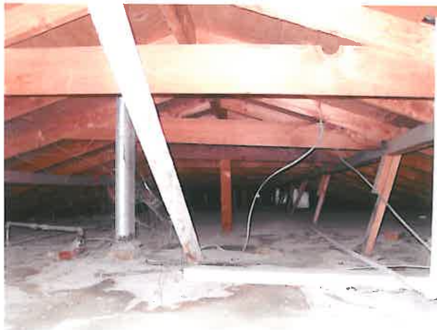
Picture 4: View of roof felt observed from east attic hatch, South Building (ACM).
