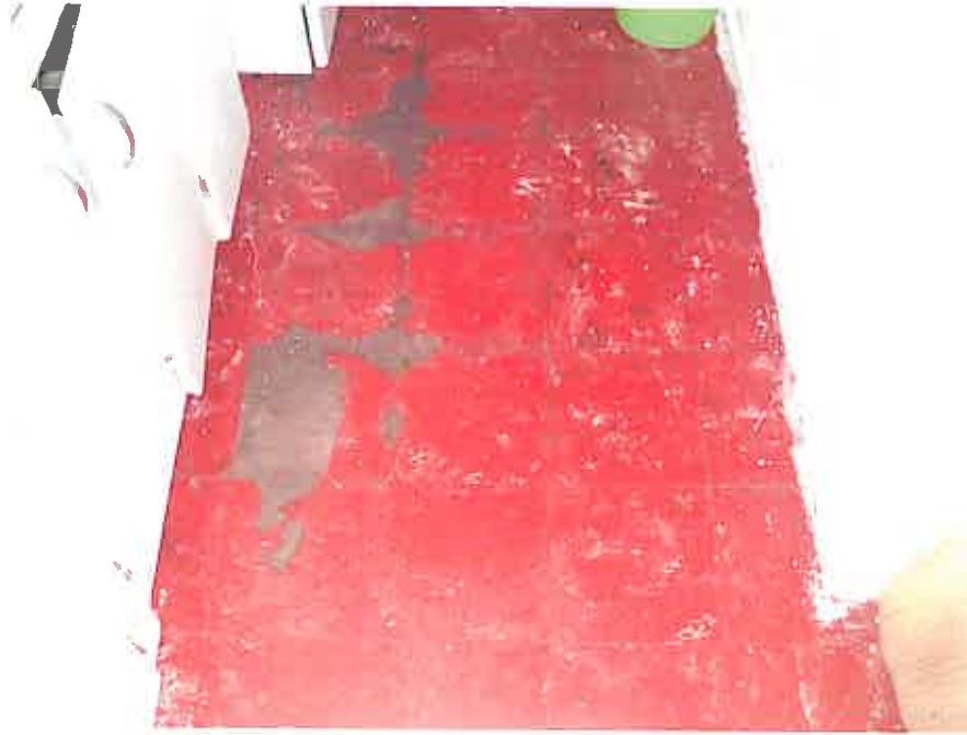
Picture 3: View of 9 X 9 red VFT (ACM) – Unit 1240 Kitchen area.
