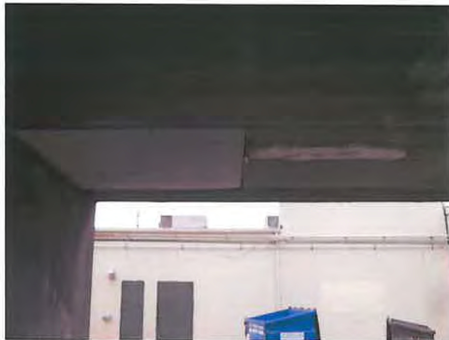
Picture 4: View of drywall and joint compound ceilings (parking area; ACCM).
