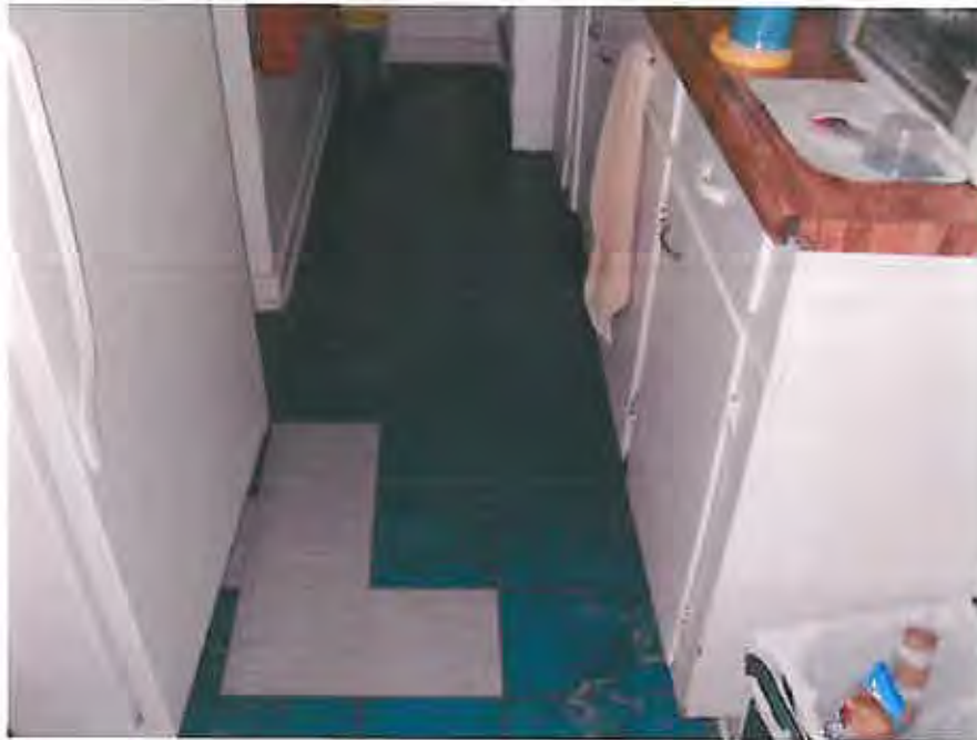
Picture 2: View of 9 X 9 blue VFT (ACM) – Unit 1242 Kitchen area.
