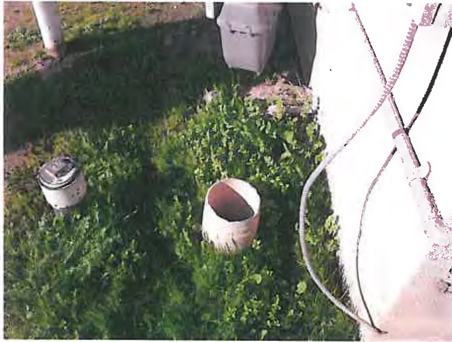
Picture 1: View of the transite pipe outside the west wall of the south building (ACM).
