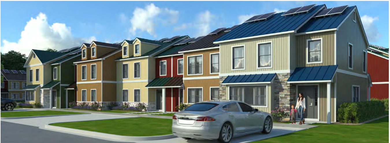
Street View of Typical Townhouse Building
